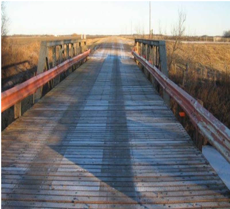
RM of Dauphin - Henderson Bridge
