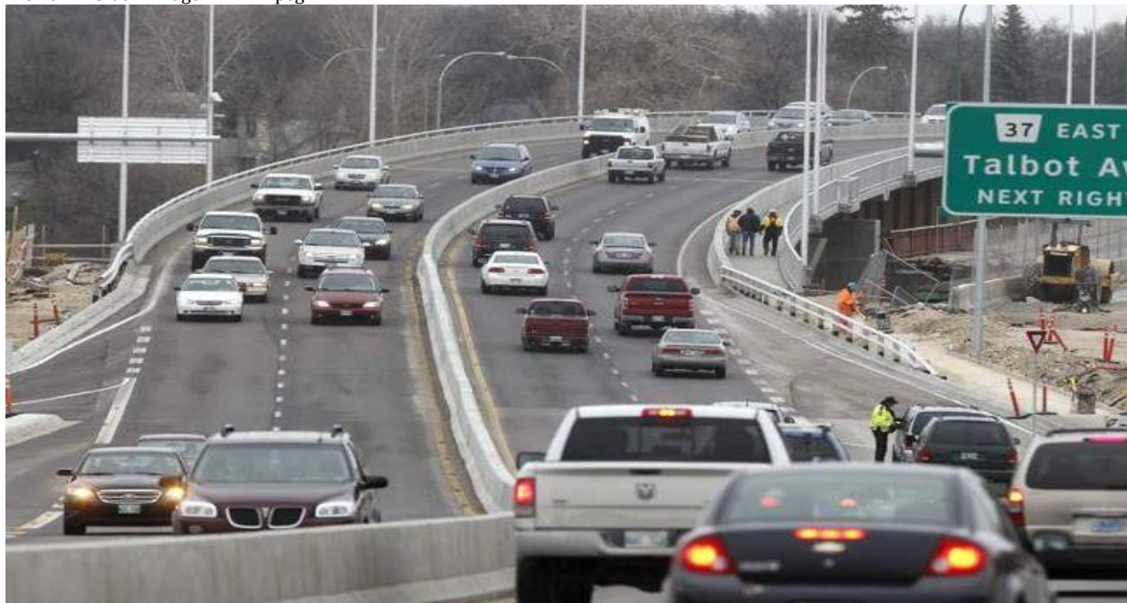
The new Disraeli Bridge in Winnipeg
