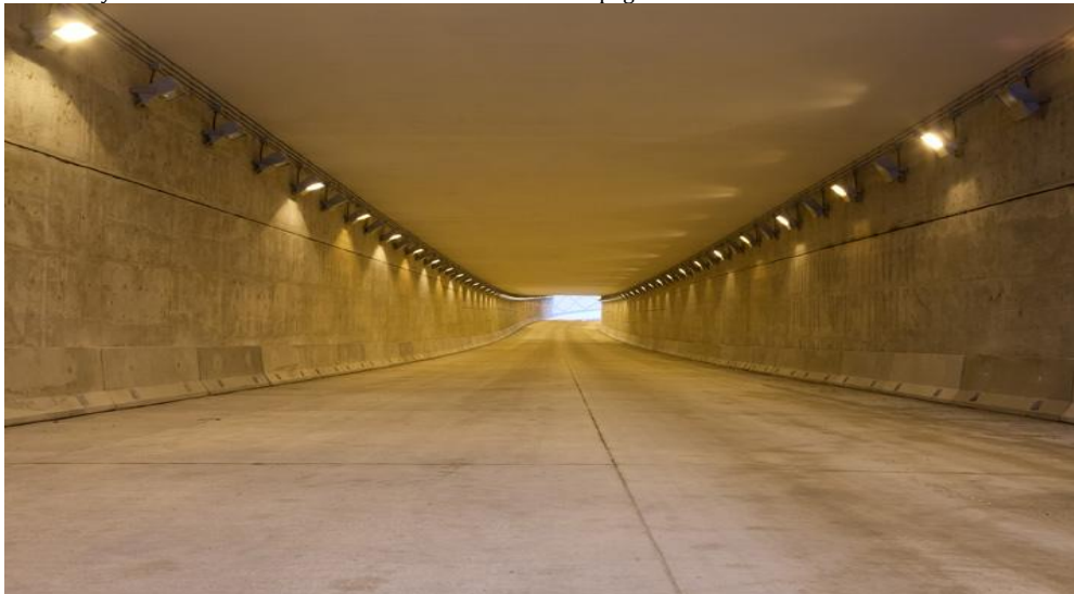
Transitway tunnel underneath the CN rail main line in Winnipeg
