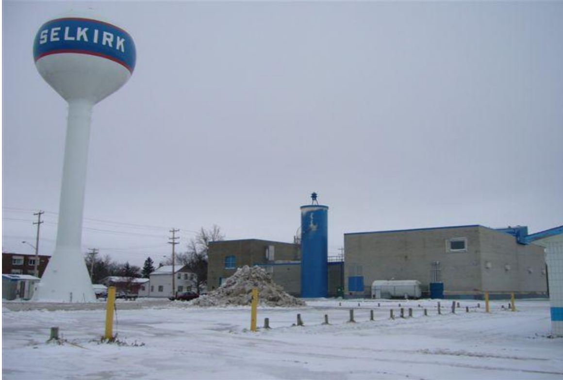
Selkirk Water Treatment Plant expansion
