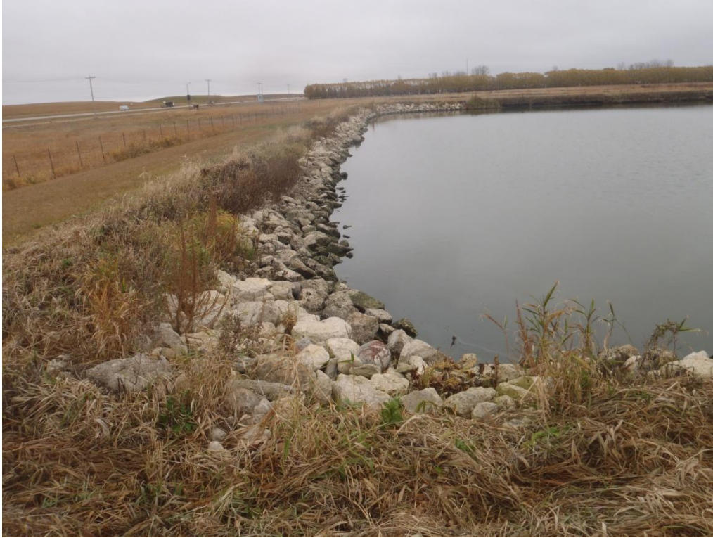
Photo 1: Existing rip rap stone on west slope of primary cell
