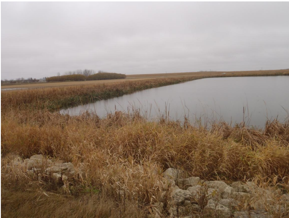
Photo 4: Vegetation growth on slopes of Secondary Cell #2
