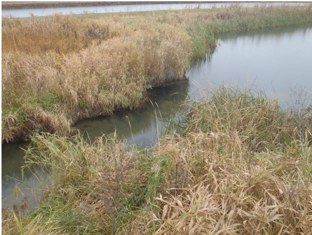
Photo 6: Portion of dike removed between Secondary Cells #1 and #2
