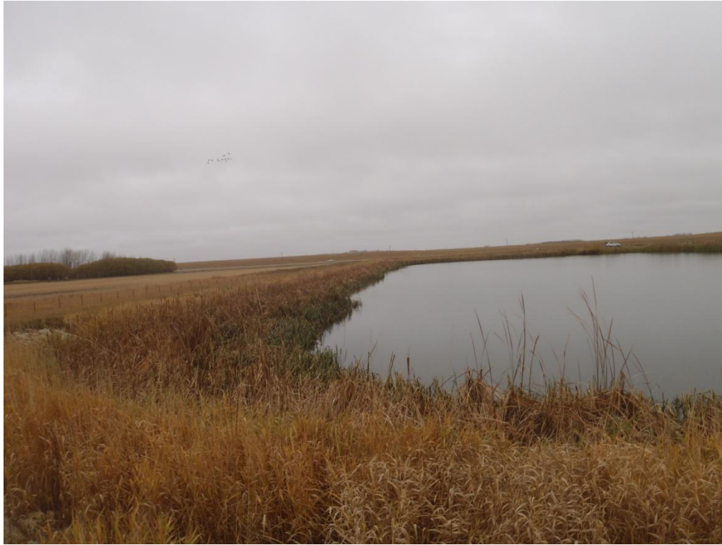
Photo 5: Vegetation growth on slopes of Secondary Cell #1
