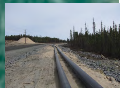
Fresh Water and Wastewater Pipelines
