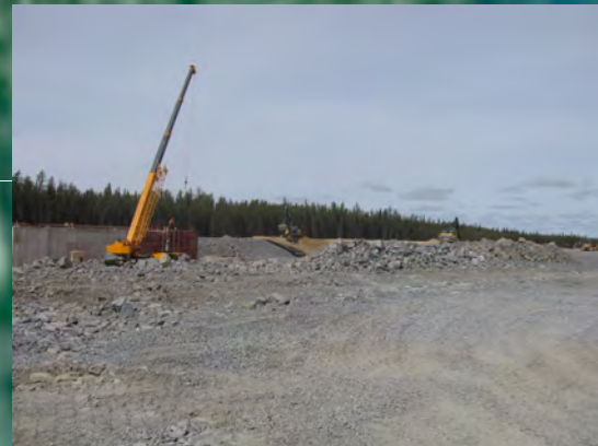
Polishing Pond Construction
