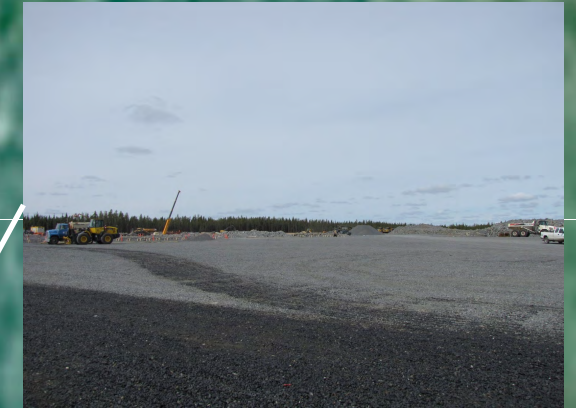
Leveled site- construction in progress
