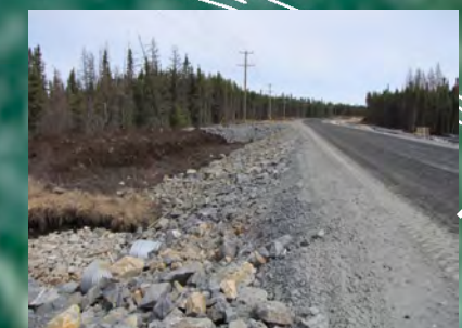
Access Road and Power Lines
