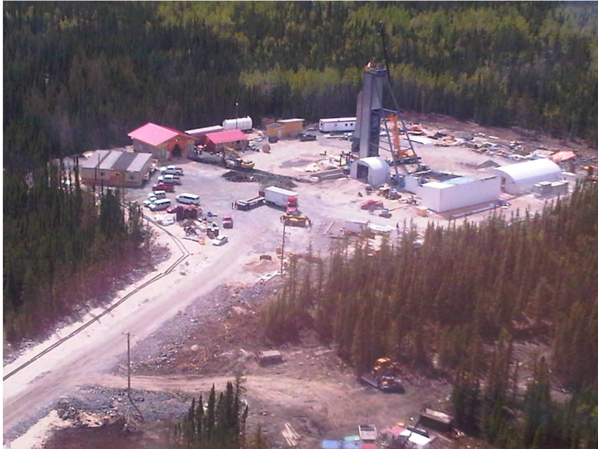
Ventilation shaft (Looking South)
