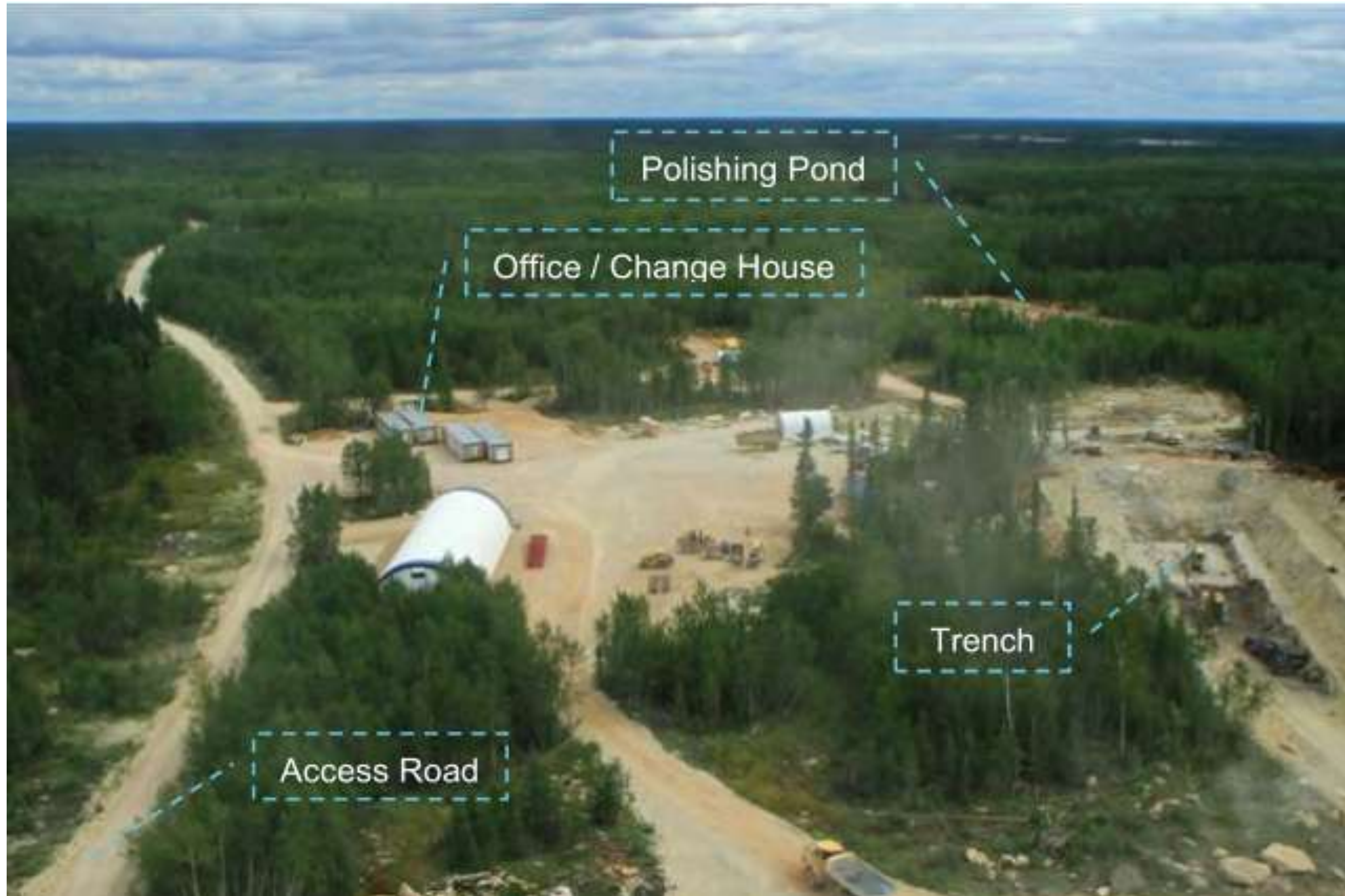
Reed AEP Site under Development, looking east (August 2012)
