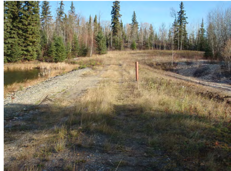
Monitoring well at existing Anderson Dam
