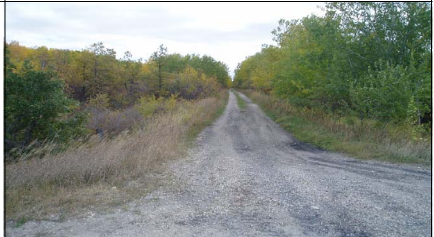
Decommissioned rail bed at Road 32 E looking southeast.
