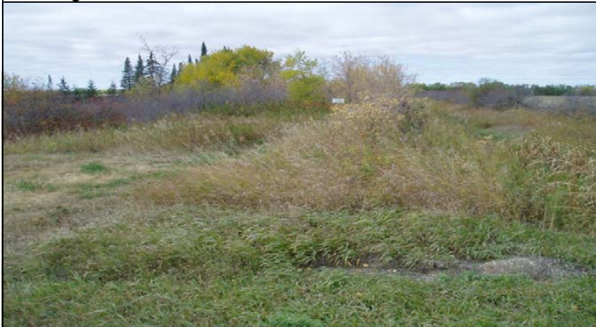
Decommissioned rail bed at Briercliff Road looking northwest.
