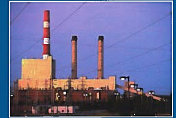
345 MW C 1958 (1st stage) C 2002 (CT's)
