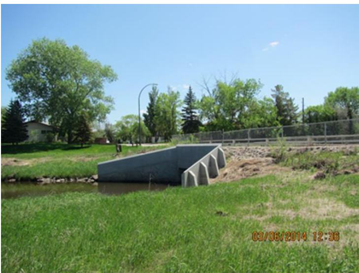
Figure 2.1 Existing Culvert on Ness Avenue at Sturgeon Creek
