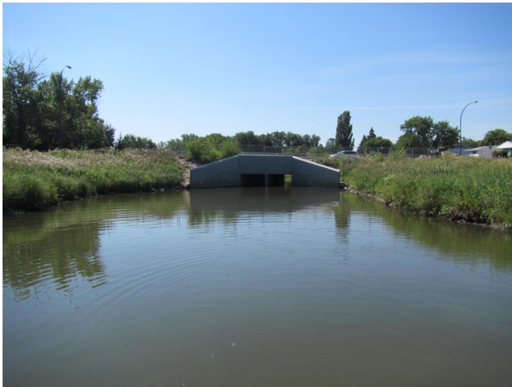
Photo No. 2 Upstream side of Ness Avenue Crossing – August 13, 2014
