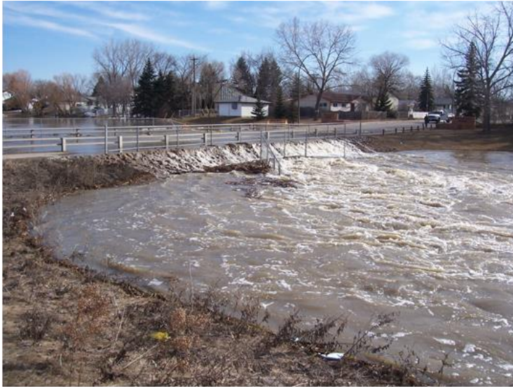
Figure 2.2 Overflow on Ness Avenue at Sturgeon Creek during spring freshet.
