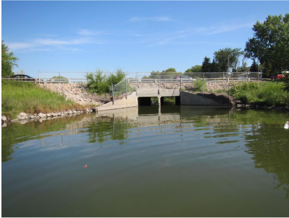
Photo No. 3 Downstream side of Ness Avenue Crossing – August 13, 2014
