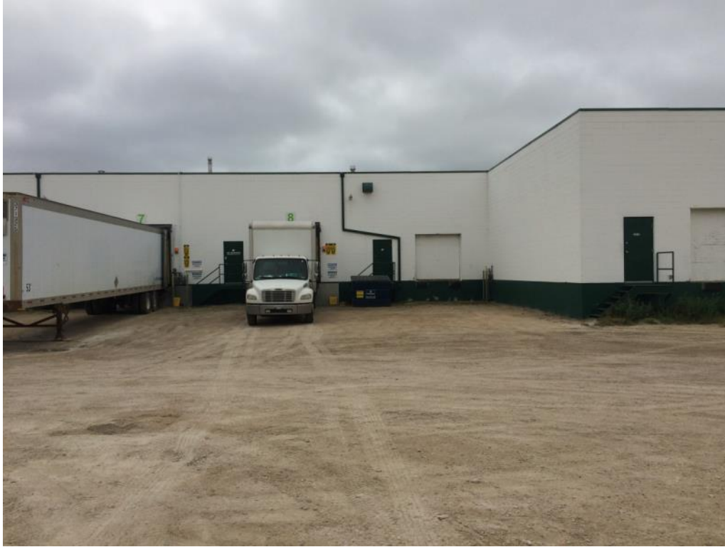
Photo 3-5: Looking south to warehouse across common drive through.
