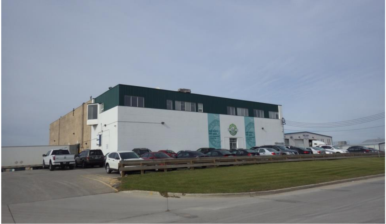
Photo 1-3: Looking at processing plant and general office at 69 Eagle Drive.
