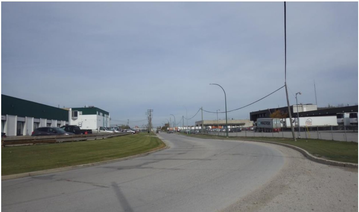
Photo 5-4: Looking north along Eagle Drive to processing plant (left side).
