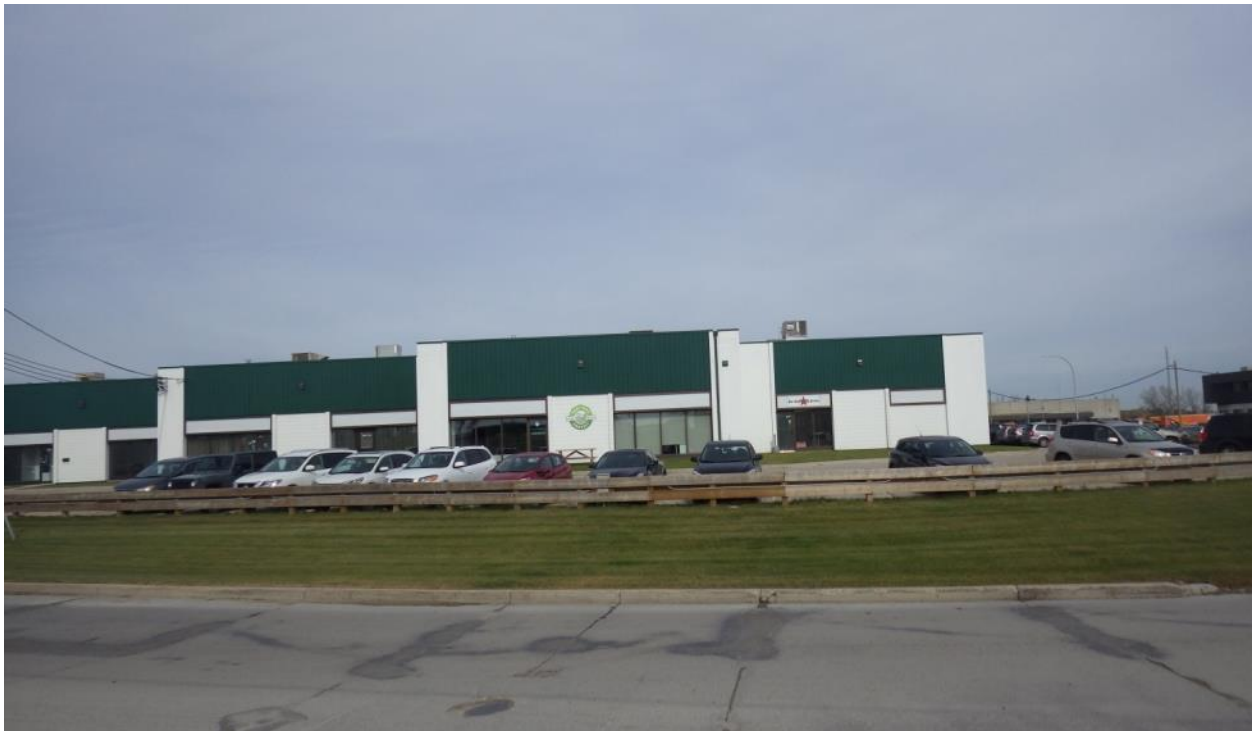
Photo 1-4: Customer Office at 79 Eagle Drive.
