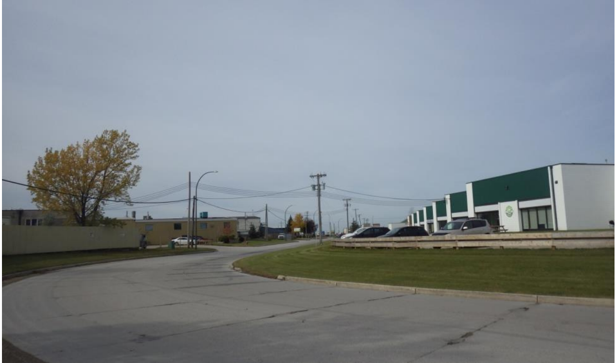
Photo 5-3: Looking west along Eagle Drive and subject property (Unit 210-79 Eagle Drive at right).
