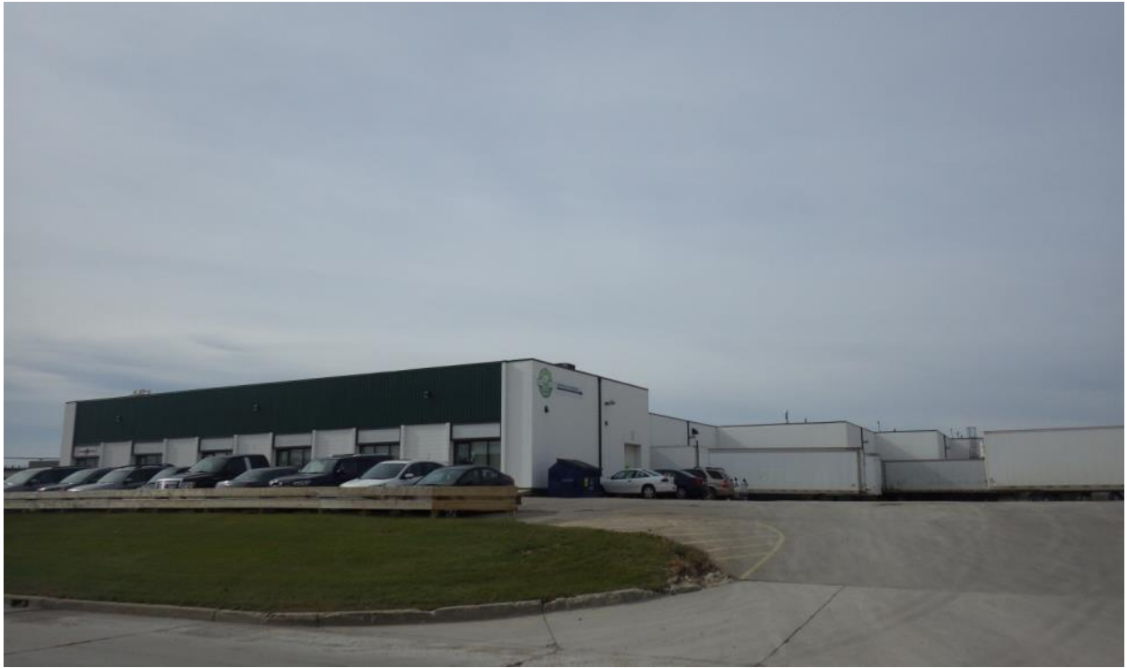
Photo 1-1: Looking to warehouse at 79 Eagle Drive.
