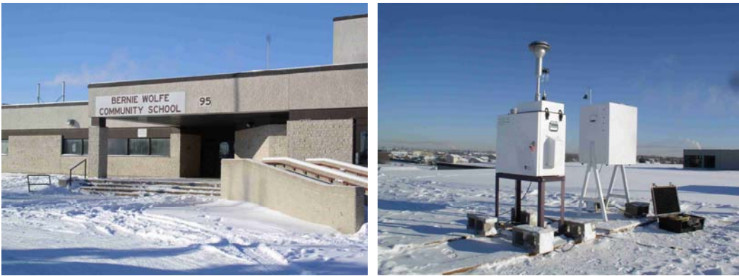
Figure 6. Phase I Site: Bernie Wolfe School, 95 Bournais Drive
