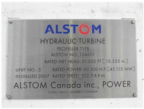
Figure 12 Unit No. 5 Nameplate Post Refurbishment, 2007
