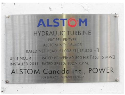
Figure 11 Unit No. 4 Nameplate Post Refurbishment, 2011
