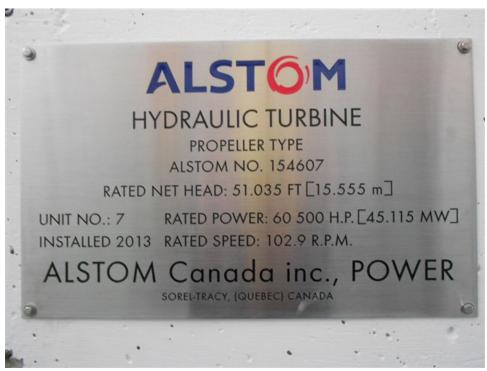
Figure 14 Unit No. 7 Nameplate Post Refurbishment, 2013
