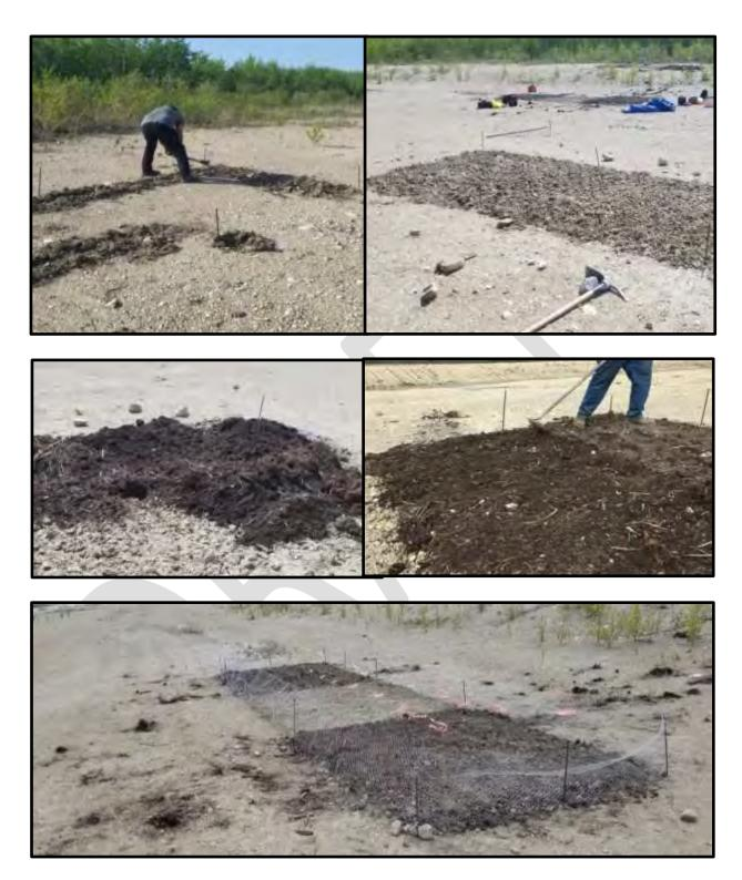
**Photo Array 2**: Trial Set-up (June 3<sup>rd</sup> and 4<sup>th</sup>, 2019) – Plots were decompacted to 0.30m using a pick axe; organics were dug, hauled and placed on appropriate sub-plots; organics were spread and blended into the decompacted till; animal exclusion measures were installed; grasses were seeded on following site preparation.
