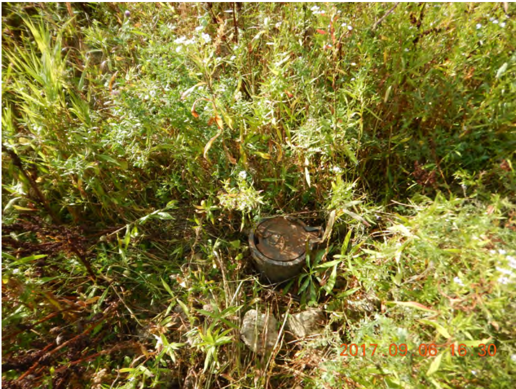
Photo 1: Low level sampling pipe steel protective casing.
