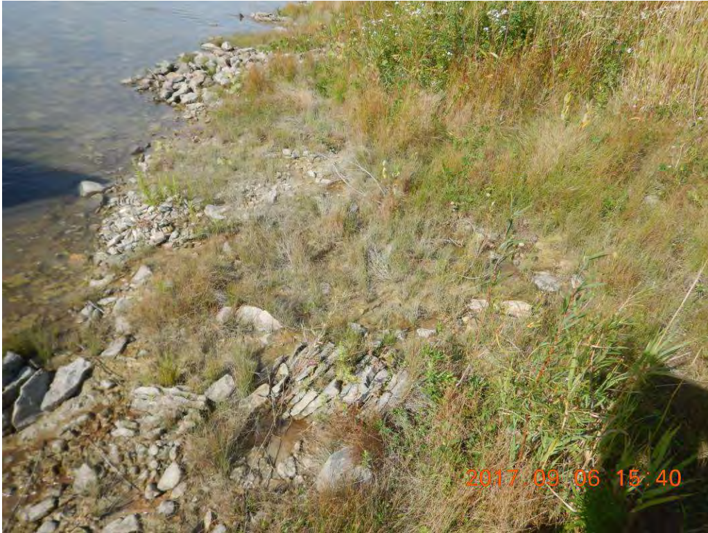
Photo 2: Tie-in of 21A2 filter drain to Low Flow Channel.
