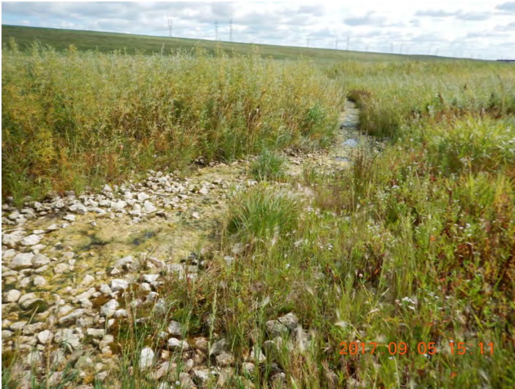
Photo 2: Discharge ditches at 7A1 effectively direct water to LFC.
