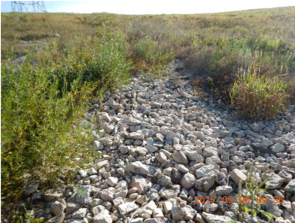
Photo 2: Water flowing through 11A2 filter and finding alternate flow paths to LFC.
