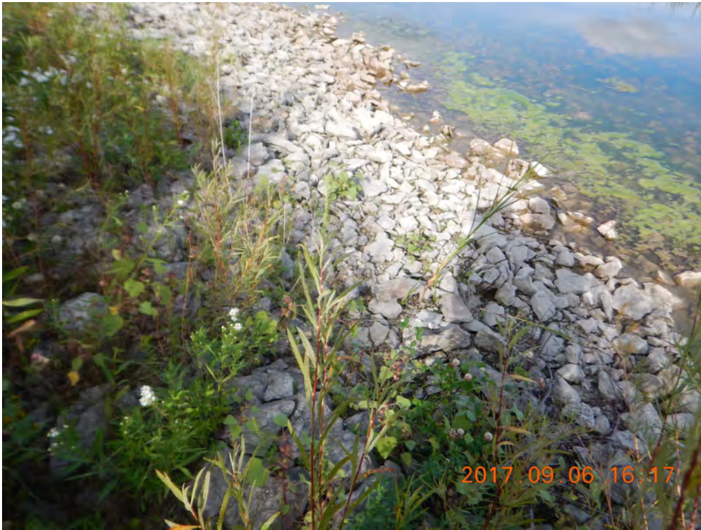
Photo 2: Tie in of discharge channel to LFC at 23A1.
