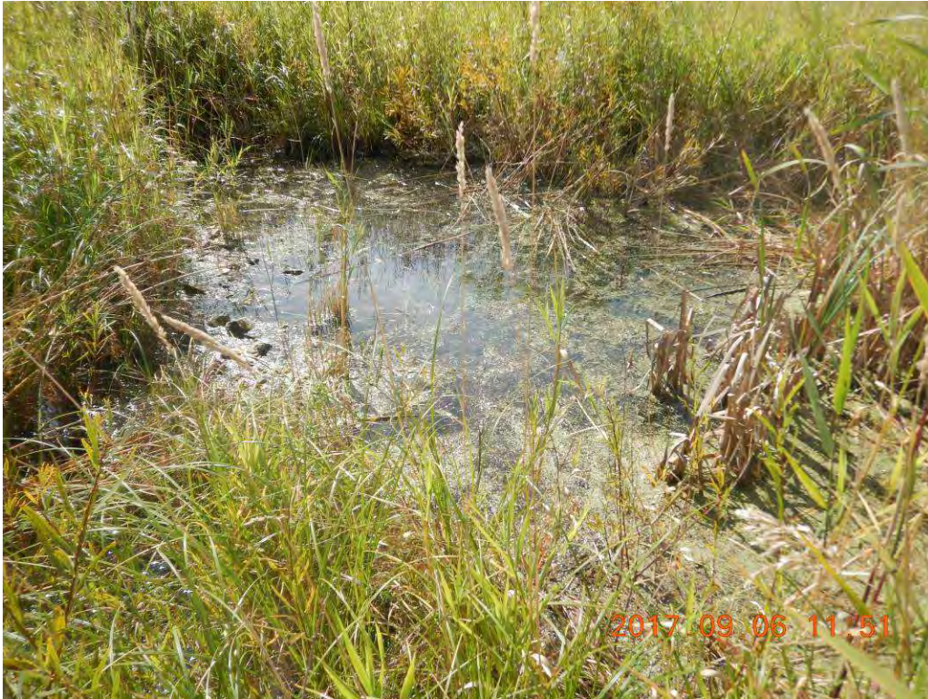
Photo 2: Water ponding beside the French drain at 17A2.
