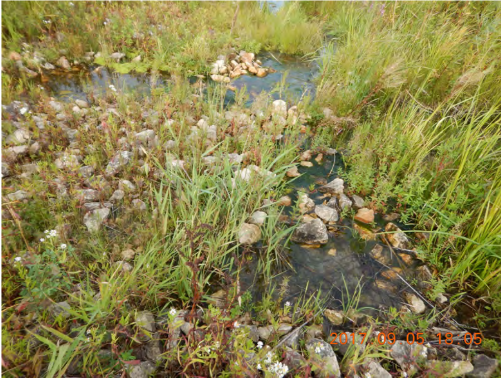
Photo 2: Water flowing through 10A1 filter and finding alternate flow paths to LFC.
