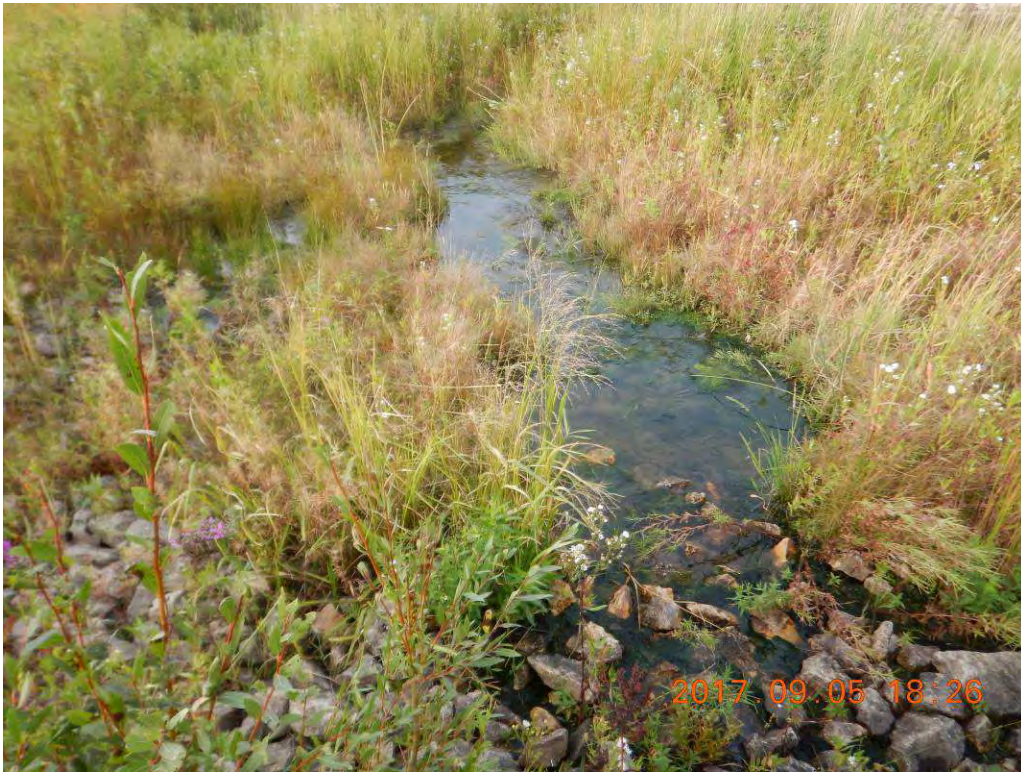
Photo 2: Water flowing through 11A1 filter and finding alternate flow path to LFC.
