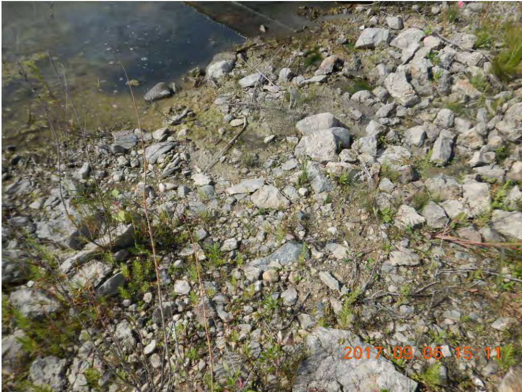
Photo 1: Tie-in of filter drain to Low Flow Channel.
