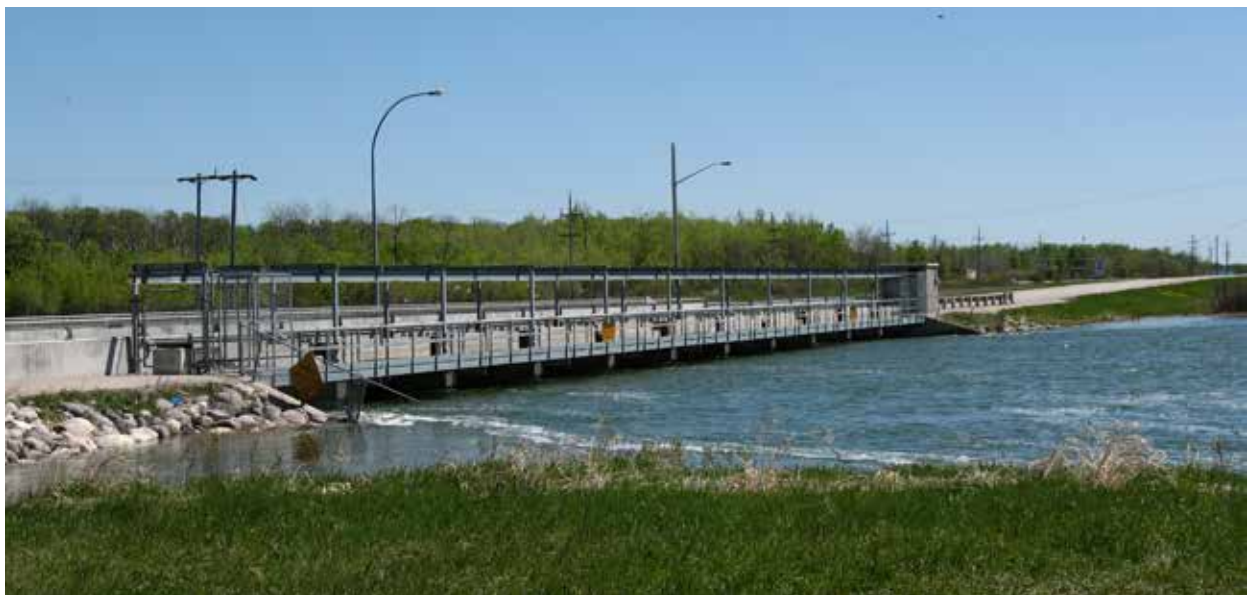
Fairford River Water Control Structure
