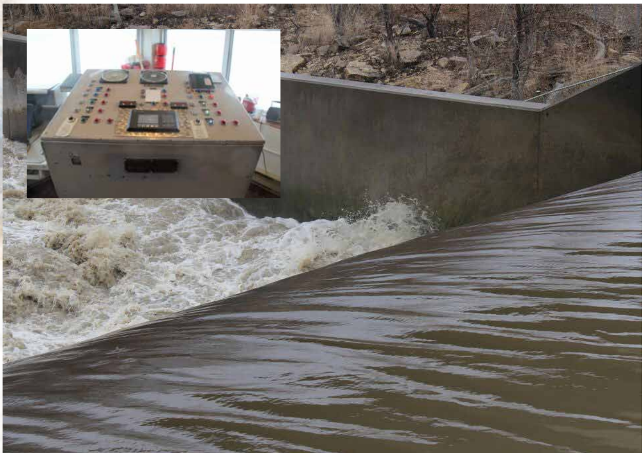
Portage Diversion and Control Panel Inside the Operations Room
