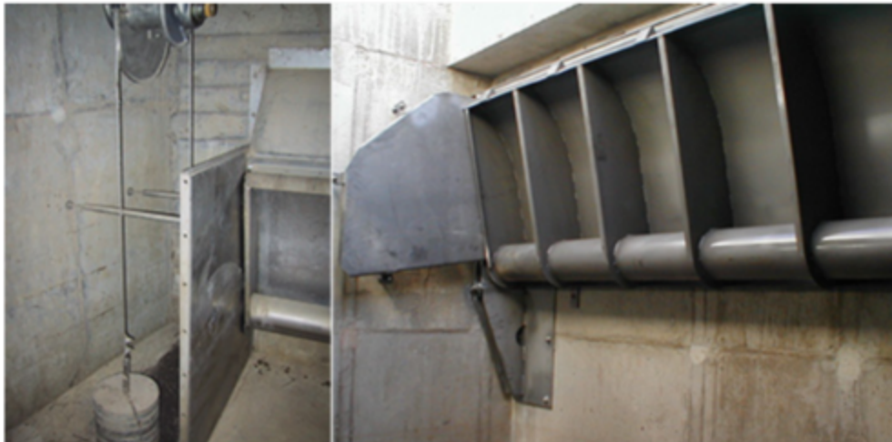
Figure 4-1. Examples of TRU-BEND Installations
