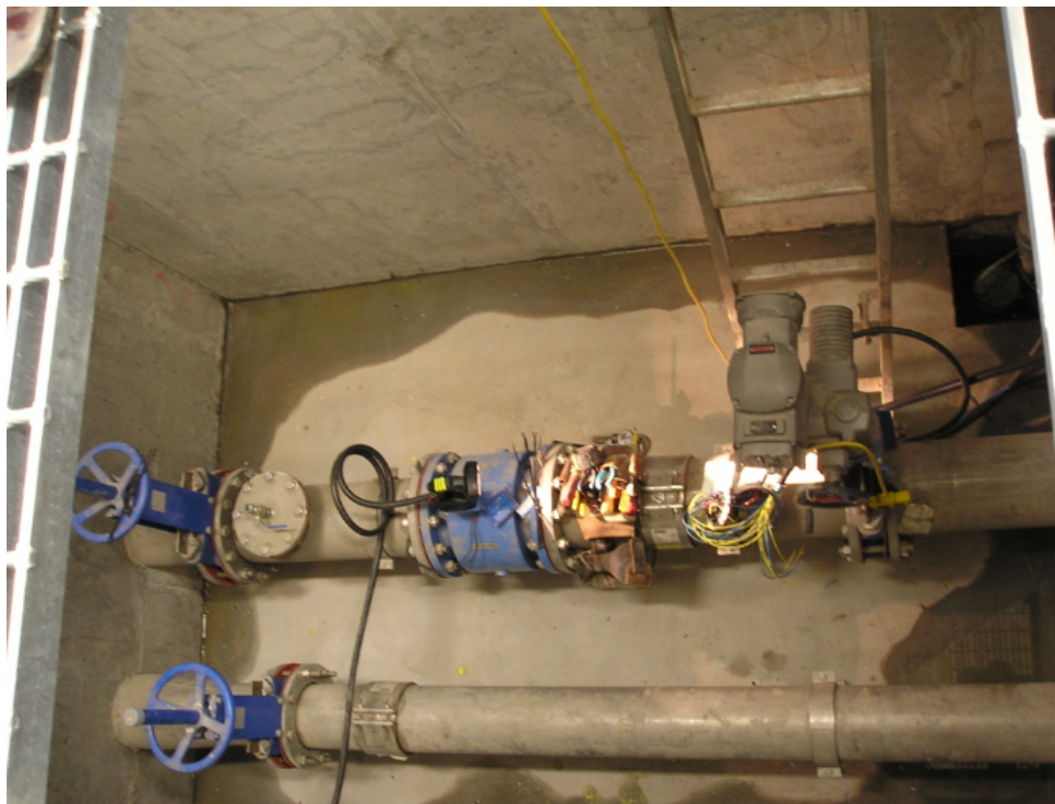
Figure 6-1. Example of HYDROVEX® FluidMIDu Installation
