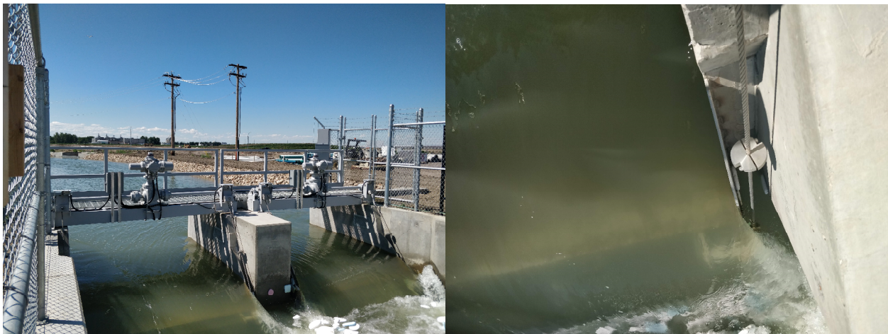
Figure 4-2. Example of Instream’s Downward Opening Gate Installation (Picture credit: Instream Water Control Projects Ltd.)
