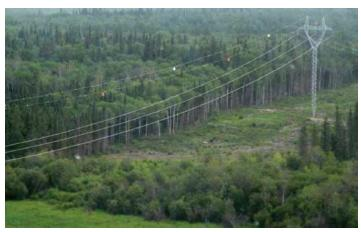
Photo 15: Bird Diverters on a Transmission Line
