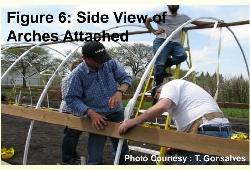
Random lengths of 2x6 were bolted to the inside of the arches 3' above where the foot is attached to the plate (Fig #6). Four foot lengths of 2x4 (Fig # 7). were bolted into the holes This provides "lateral strength".
