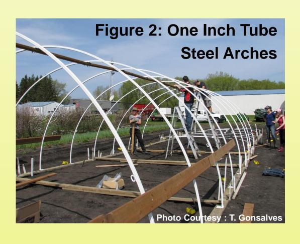
• The choice was made to use 1" tube steel for the arches (Fig #2).
