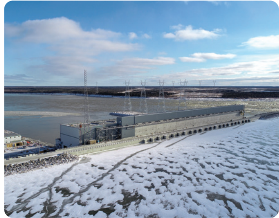
Keeyask generating station
