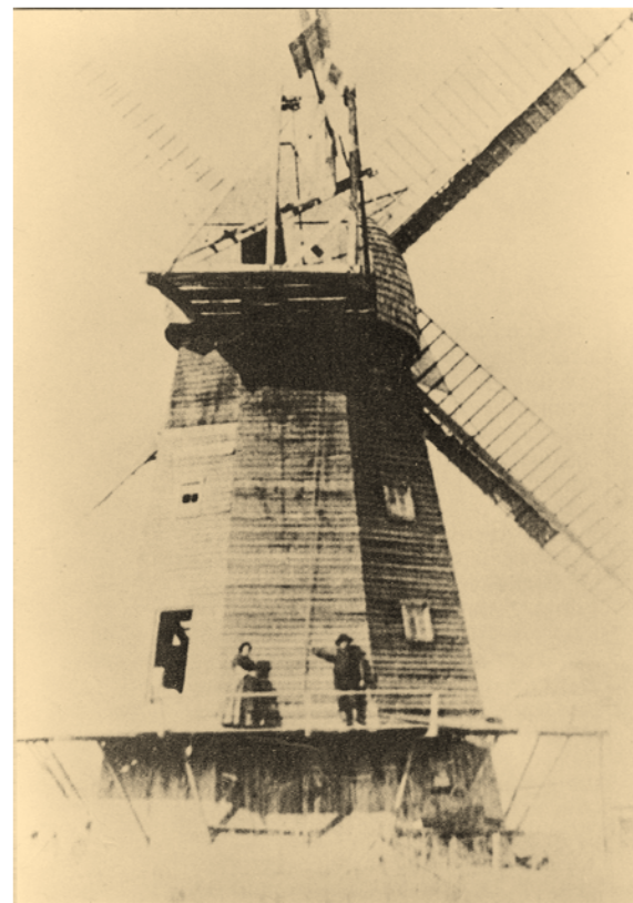
Figure 6 The Reinland windmill, one of the early landmarks in the West Reserve. Constructed by Johann Bergman in 1878-79, it was used for grinding wheat and crushing feed until it was dismantled at the turn of the century. (Reinland, 1976: 53)
