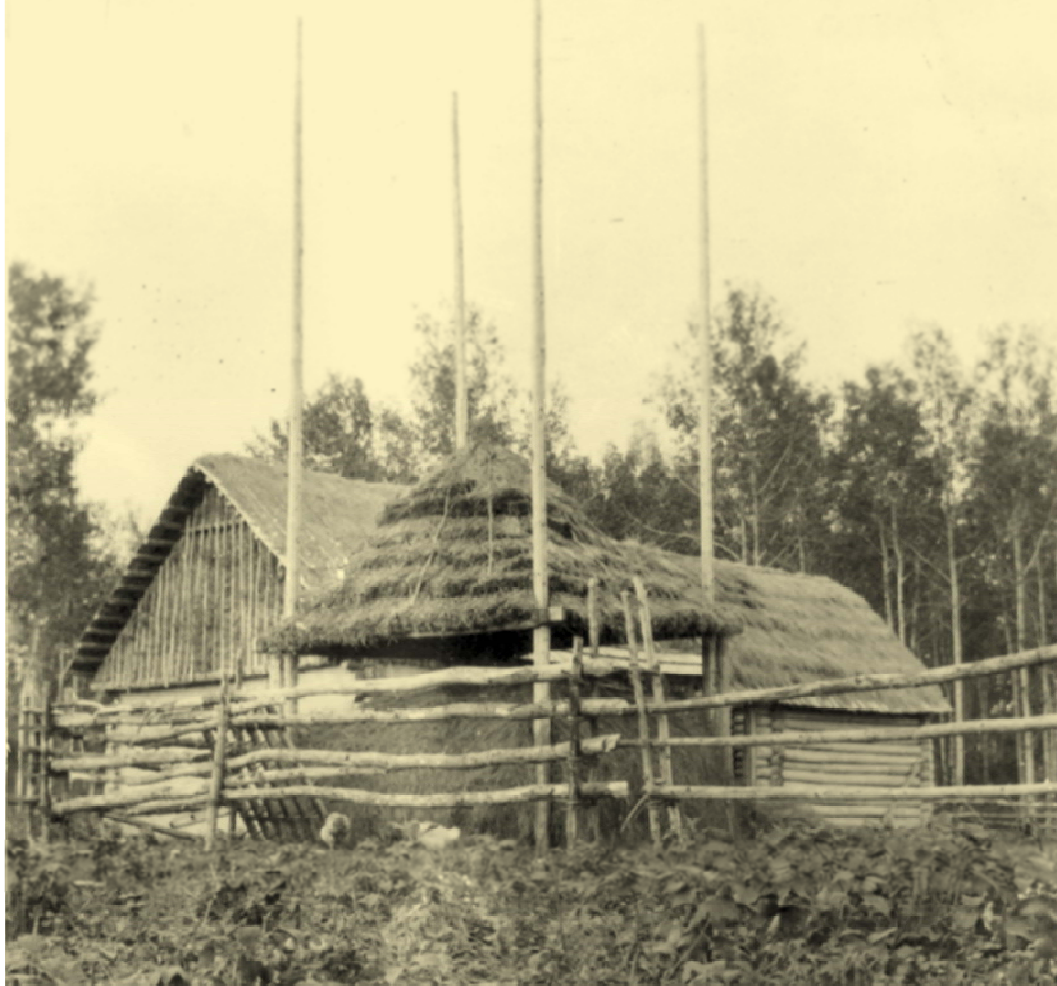
Figure 23 Early log barn in the Foley area. Feed hay was stored under the thatch-roofed structure in the foreground. (Provincial Archives Manitoba)
