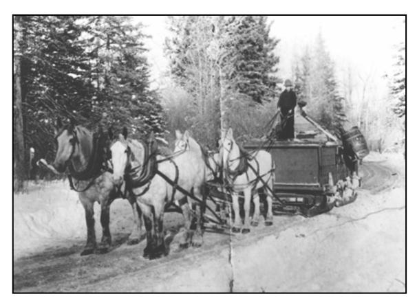
Water sleigh used to create the ice roads used in lumber camps, c. 1906. Source: P.A.M.
