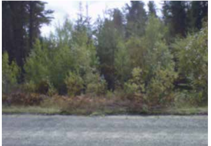
Figure 6 - Forestry road post-decommissioning after twenty years.
