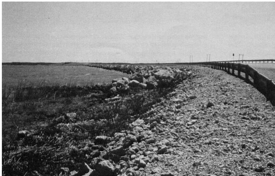
Figure 6 Cat Head dolomite in large blocks of riprap protecting the causeway along the road to Hecla Island (replacing the 'ferry route' shown in Map ER85-1-1).
