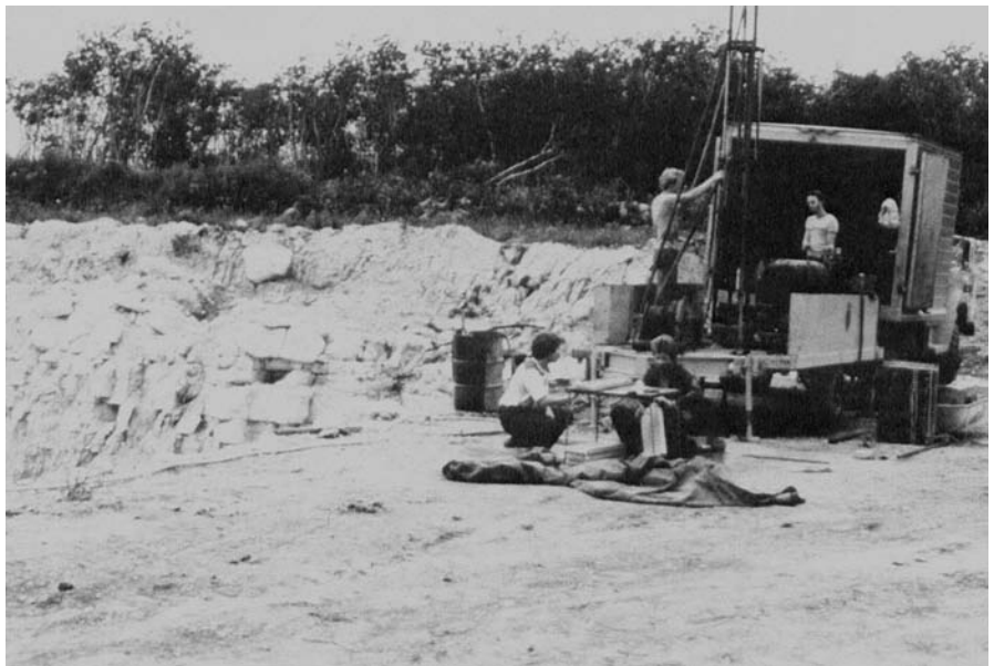
Figure 9: Geological Services drill in operation at the edge of the Winnipeg Beach quarry, in dolomitized Selkirk Member.
