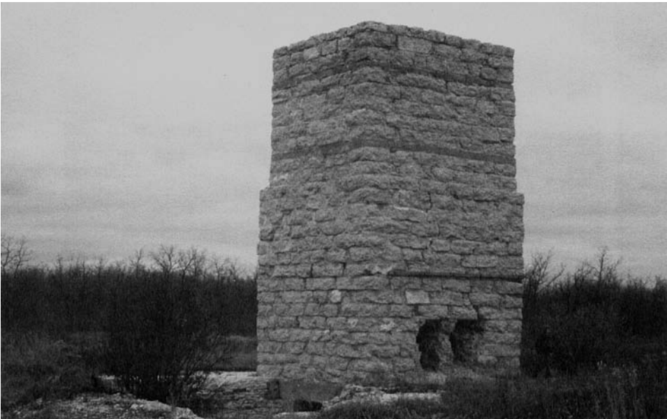
Figure 21: Oldkiln at the Birse quarry, built from one thick bed of vuggy dolomite exposed at the top of the quarry; Gun-ton Member, Stony Mountain Formation. An extensive quarry has been operated by Mulder Brothers Limited since 1982 to the northwest of the kiln.
