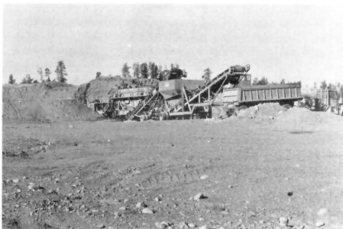
PLATE 16B: Crushing and screening of gravel from B45W2 for Department of Highways contract.
