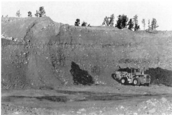
PLATE 16A: Equipment excavating gravel from B45W2 for Department of Highways contract.
