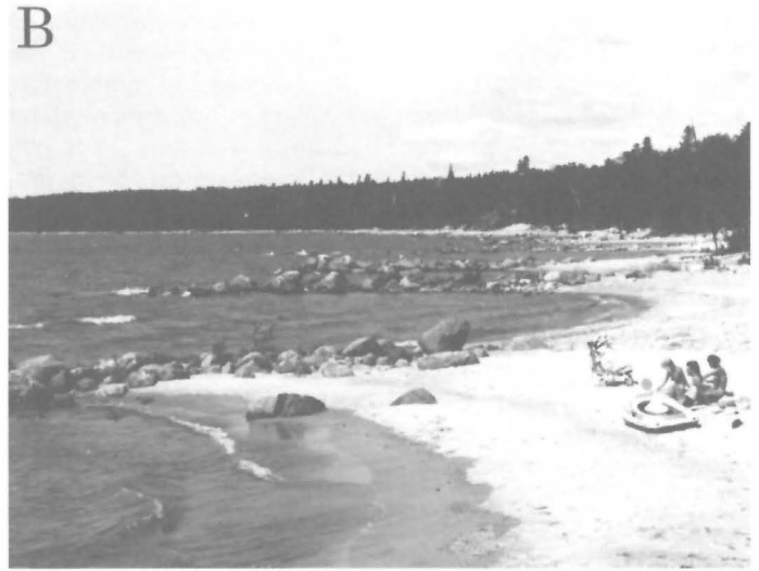
Figure 10: (A) Sea-wall at Matlock, and (B) groynes at Balsam Bay constructed to halt shoreline erosion.
