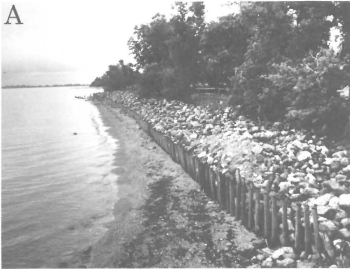
Figure 10: (A) Sea-wall at Matlock, and (B) groynes at Balsam Bay constructed to halt shoreline erosion.
