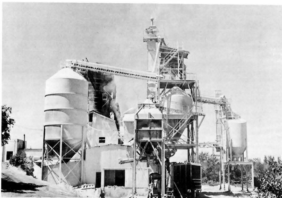
PLATE 2. Lime plant at Spearhill; Steel Brothers Canada Ltd.; lime storage bins, with kilns in background.
