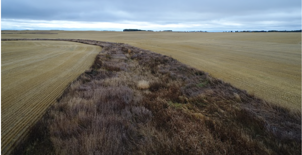
NE 13-16-17 Near Domestic Lagoon
