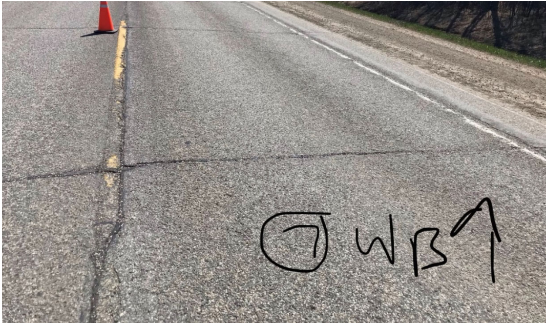
Figure 2.0.6: Transverse Cracking on PTH 23 at Carmen, Manitoba
