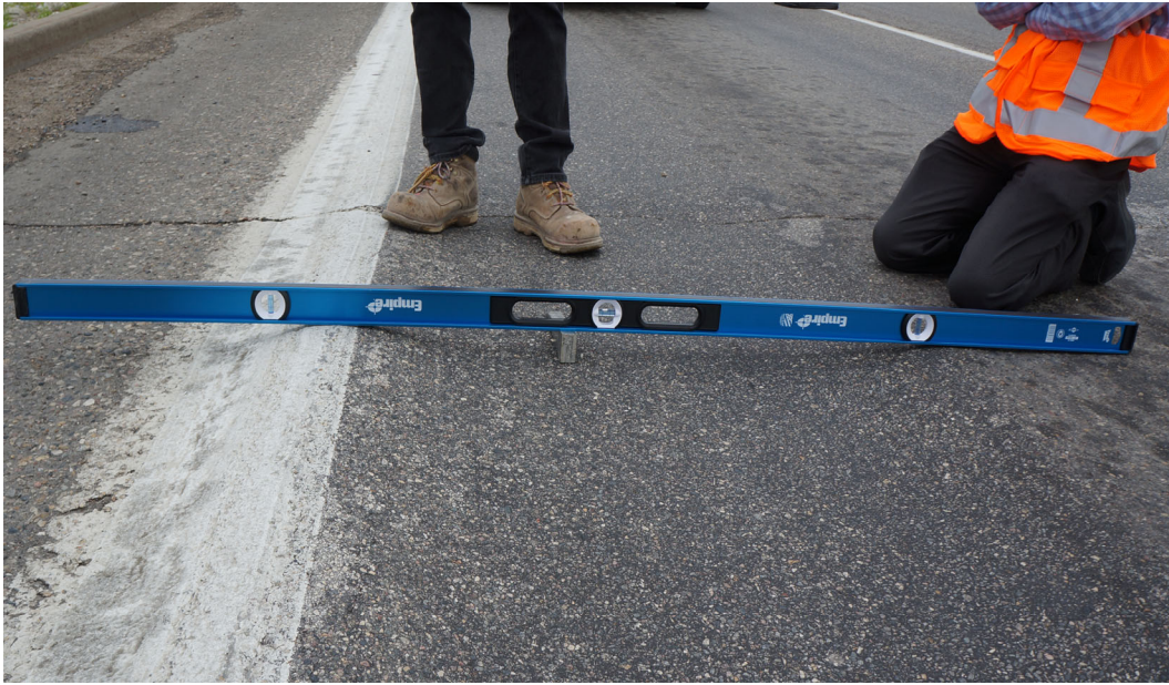
Figure 2.0.3: Surface Rutting on PTH 1 at 1st Street, Brandon, Manitoba
