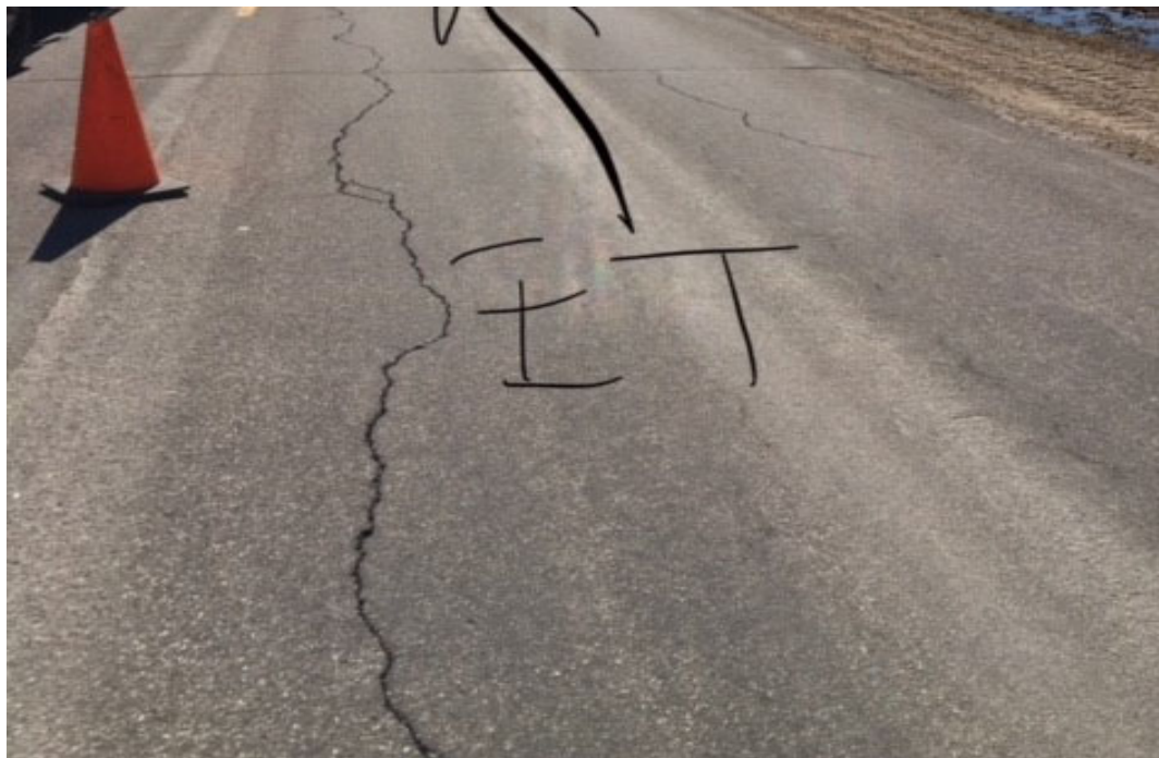
Figure 2.0.5: Longitudinal Cracking on PTH 67 at PTH 8, Manitoba
