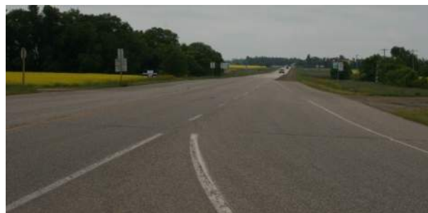
Merge taper at Service Road, south of the intersection
