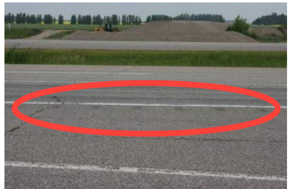
Rumble strips on the eastbound approach
