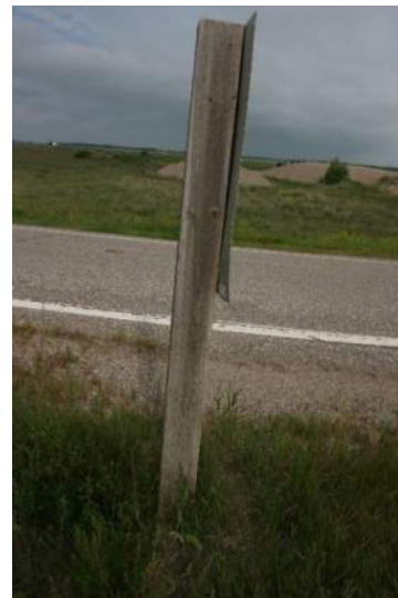
Example of Sign without shear holes
