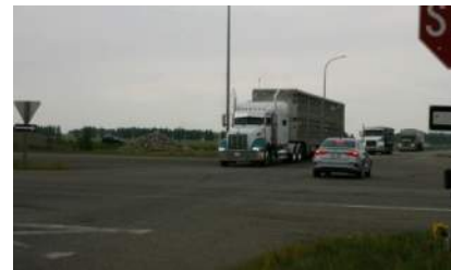
Truck and passenger vehicle crossing narrow median at same time
