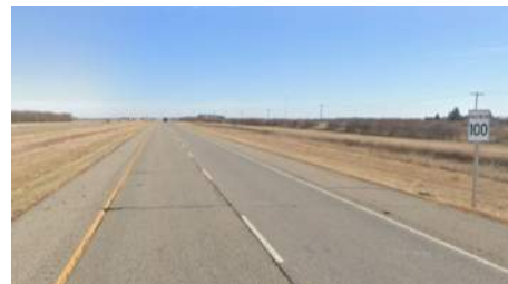
Eastbound approach single posted “Maximum 100 km/h” signage (approximately 4.0 km from intersection)
