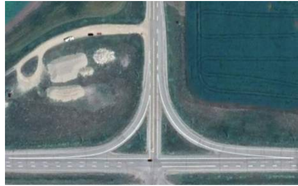
Service Road, north of intersection
