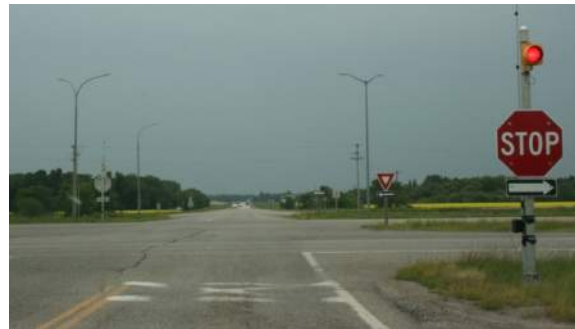
Large yield signs are located at increased offset from the travel path
