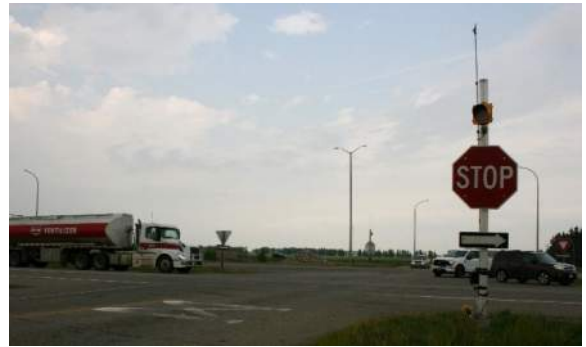
Truck waiting in the left-turn lane limits sightlines for vehicles using the median
