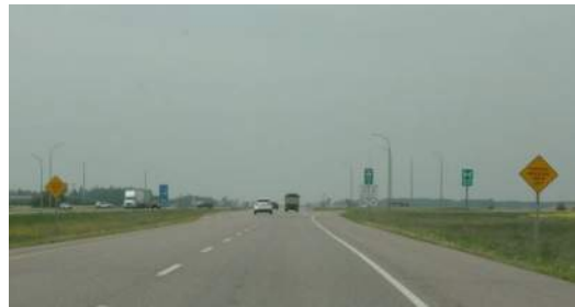
Double posted warning signs "Traffic Merging from Left" on westbound approach
