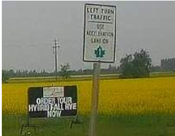
Figure 4.20: Northbound approach: Left Turning Traffic Use Acceleration Lane sign
