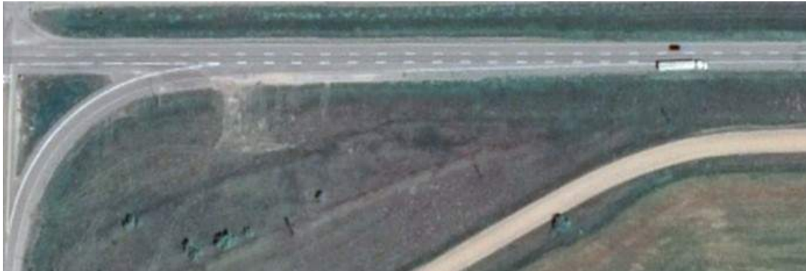
Figure 4.26: Eastbound onramp from PTH 5 to PTH 1
