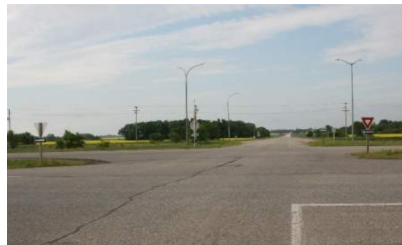
No positive guidance in the median
