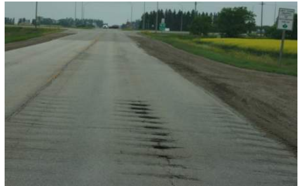
Transverse Rumble strips on the northbound approach
