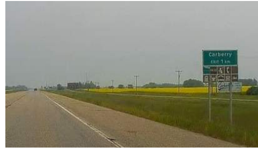
Advance destination distance sign on the eastbound approach to the intersection
