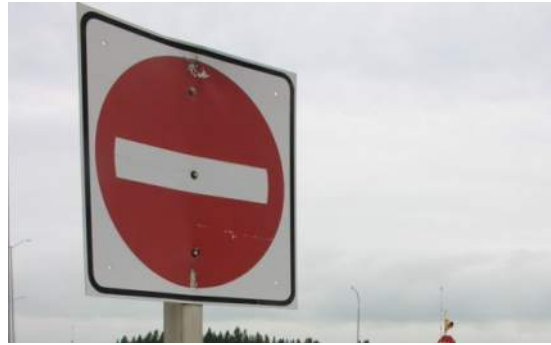
Example of Sign deterioration
