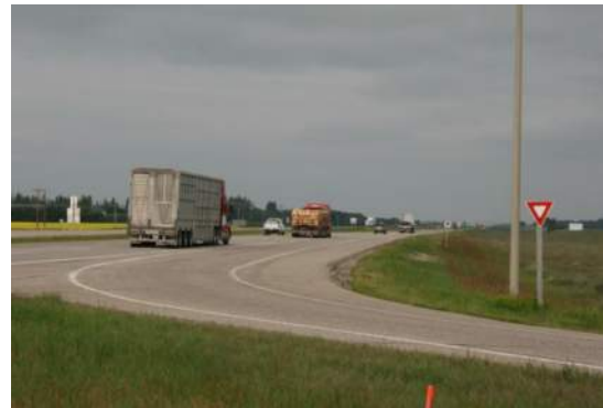
Southbound to westbound channelized right-turn lane with yield sign
