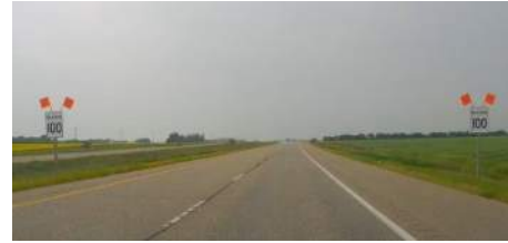
Westbound approach double posted “Maximum 100 km/h” signage
