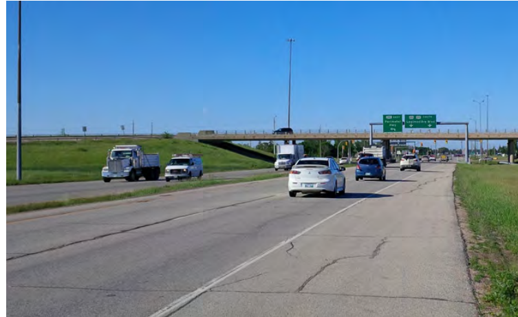
Intersection of PTH 59 and PTH 101 before construction.
