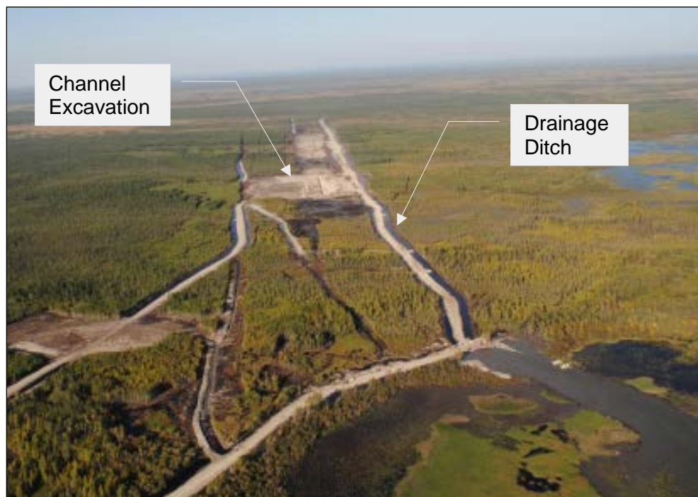
PHOTO 1 CONSTRUCTION OF REACH 1 EMERGENCY CHANNEL
