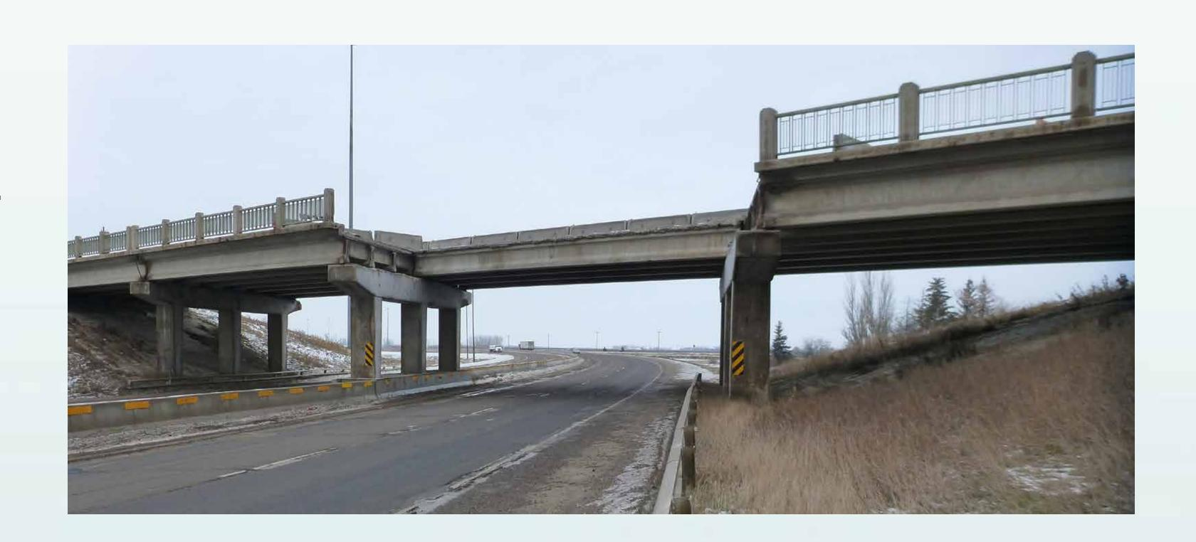
Over the years, the bridge has been damaged by several vehicle impacts, and many bridge elements are exhibiting significant deterioration. As a result, the bridge is currently restricted to a single lane.
