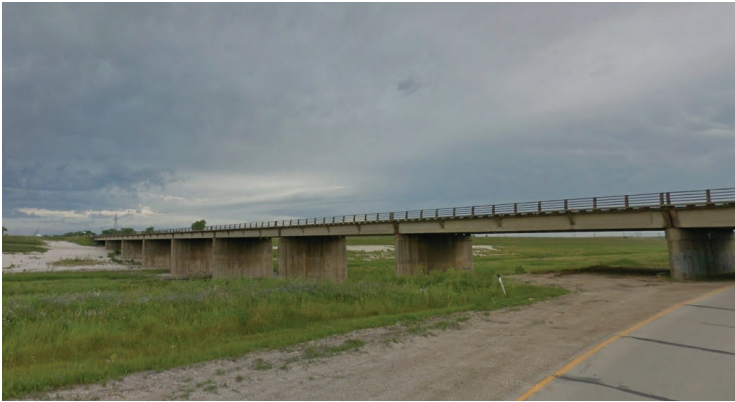
FIGURE 1 - EXISTING BRIDGE ON PTH 59
