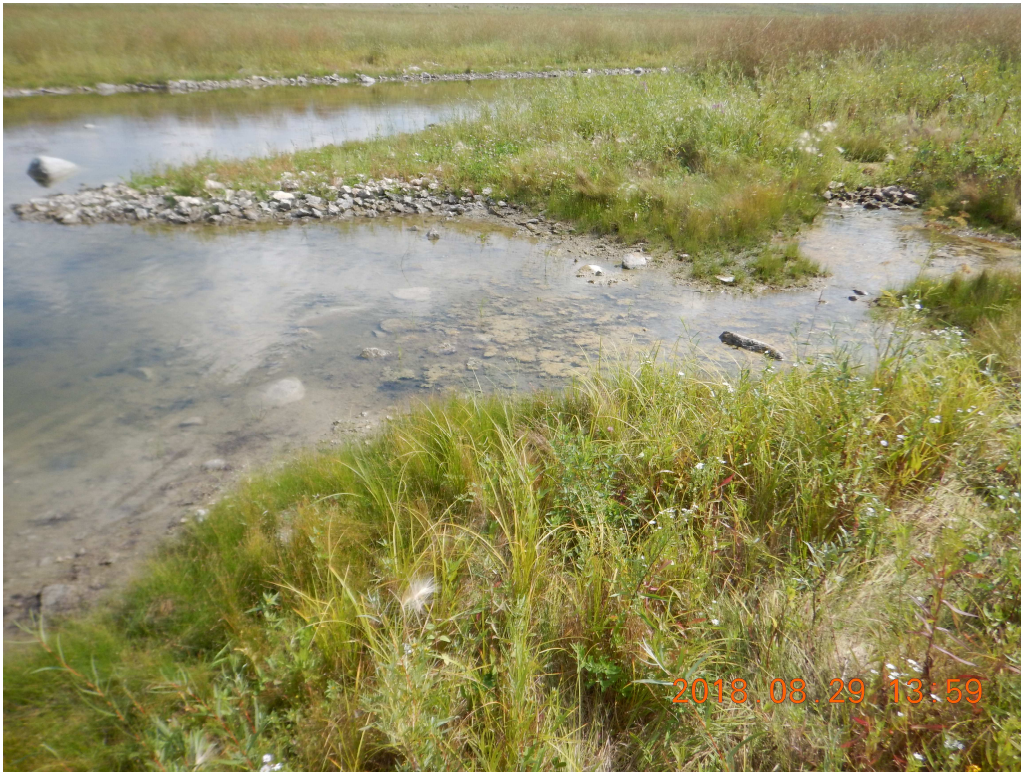
Photo 2: Water flowing through 21A1 filter and finding alternate flow path to LFC.
