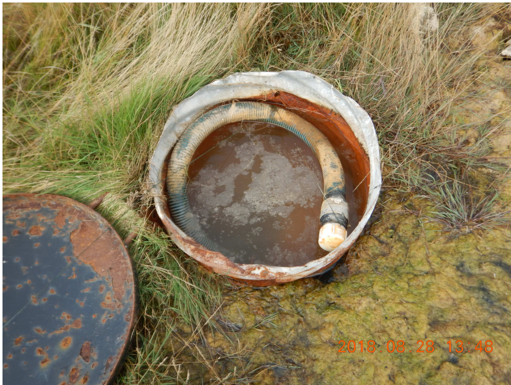
Photo 1: Low level sampling pipe and water within protective casing. MI added a new protective cap and marker to the casing after the annual inspection was conducted.
