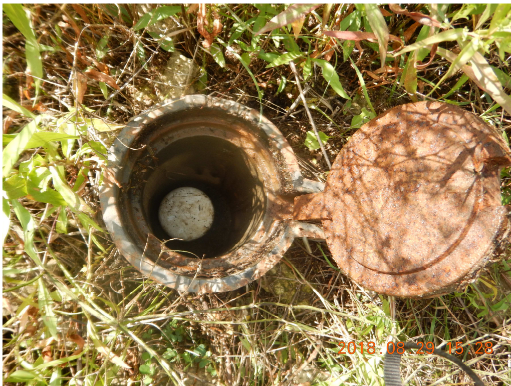
Photo 1: Low level sampling pipe steel protective casing.
