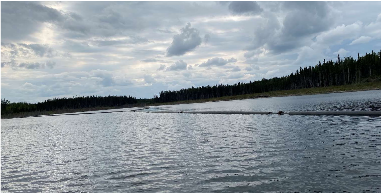
Figure 2 – Anderson TIA Upstream Inflow and Nearby Tailings Pipes
