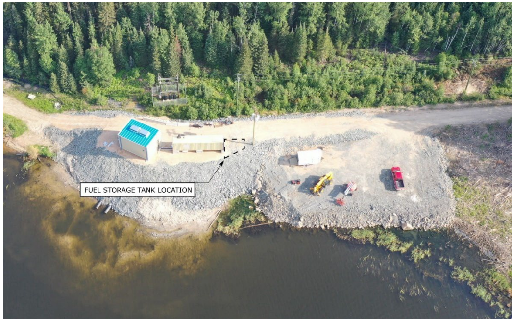
Photograph 1 – Aerial view of Anderson TIA Reclaim Pumphouse
