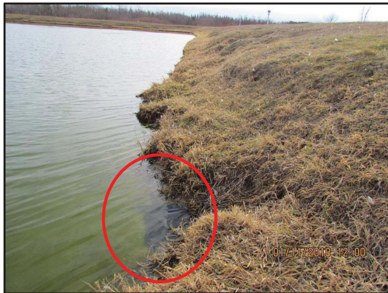
Figure 6 - Exposed liner, west secondary cell berm looking south (Source: Parks)
