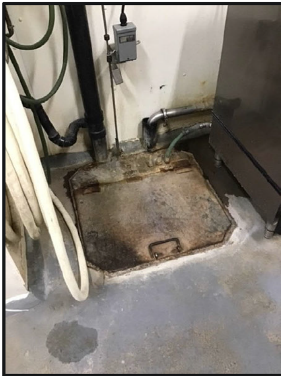
Figure 10. Receiving Bay Pit
