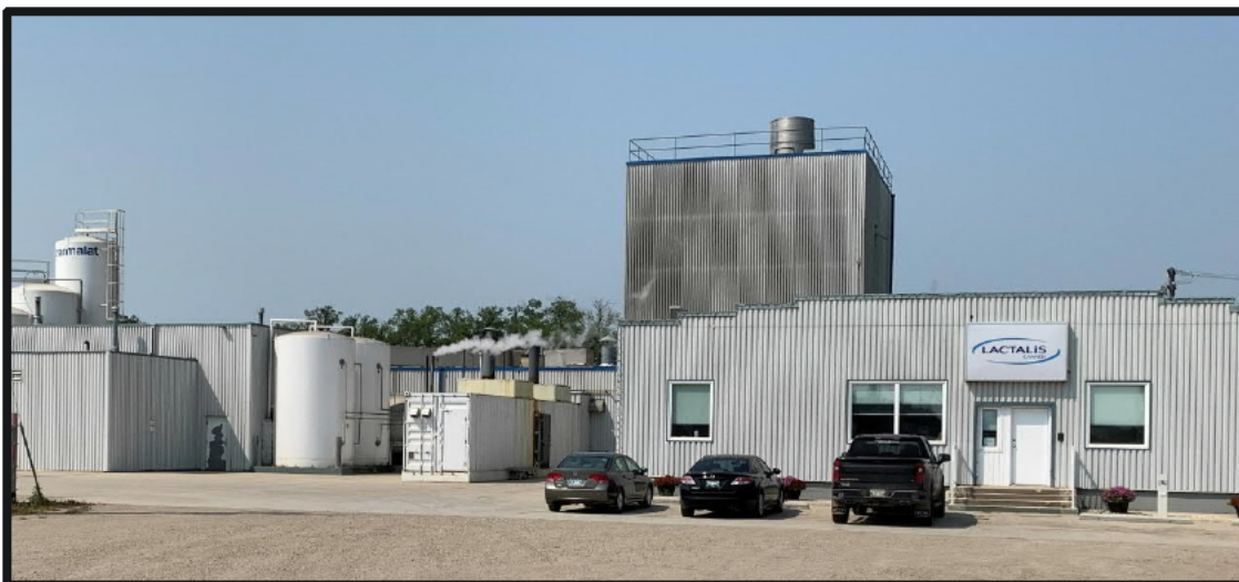
Figure 1. View of the Front of the St. Claude Facility
