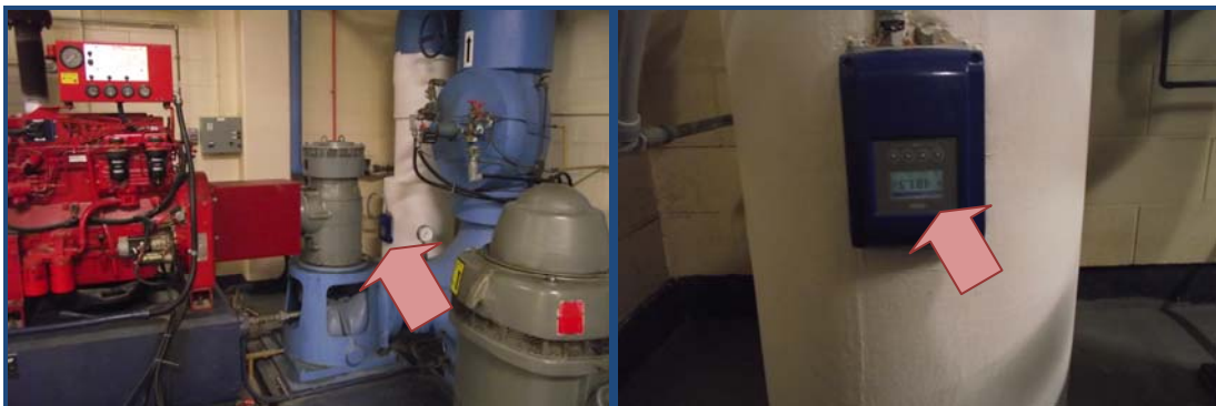
Figure 2-7 Water Plant Treated Water Distribution Meter
