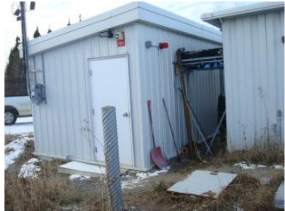
1.4 UV Building entrance and conduits to SBR building
