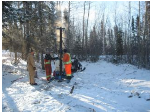
2.2 Borehole drilling (TH-12) at proposed lift station location
