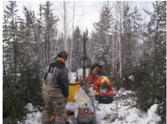
4.4 Geotechnical investigation at Test Hole TH-8
