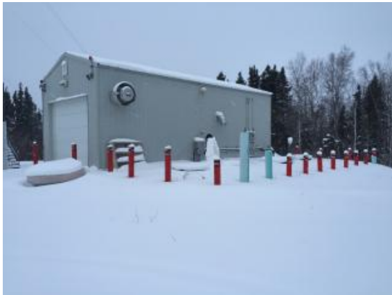
1.9 Sludge digester building
