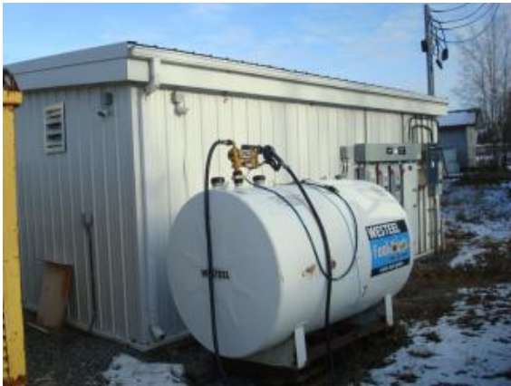
1.3 UV Building and fuel tank
