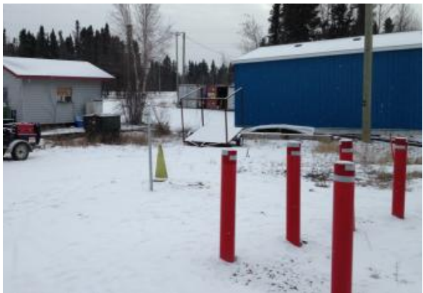
1.12 Manhole MH view from NW looking along proposed gravity sewer line route
