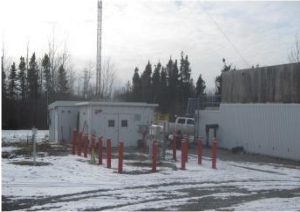
1.1 SBR building and underground transfer tank
