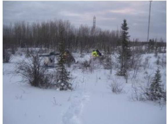
3.2 Drill rig mobilization in open area East of Lagoon Site 1
