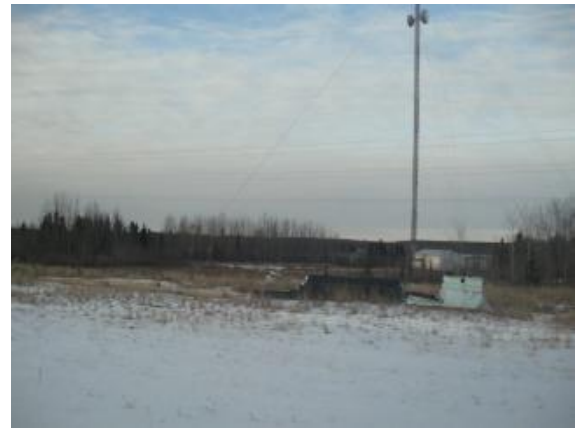
2.4 View North of Communication Tower from Probe Hole PH-19
