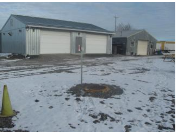
1.11 Manhole MH3 view from SW
