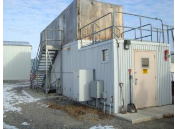
1.8 BioBrane exterior view from SW
