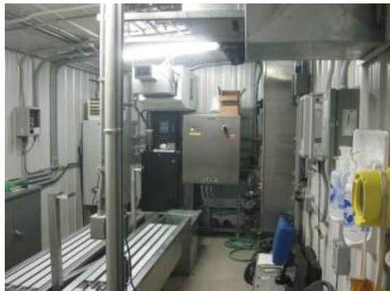
1.5 Interior of UV building
