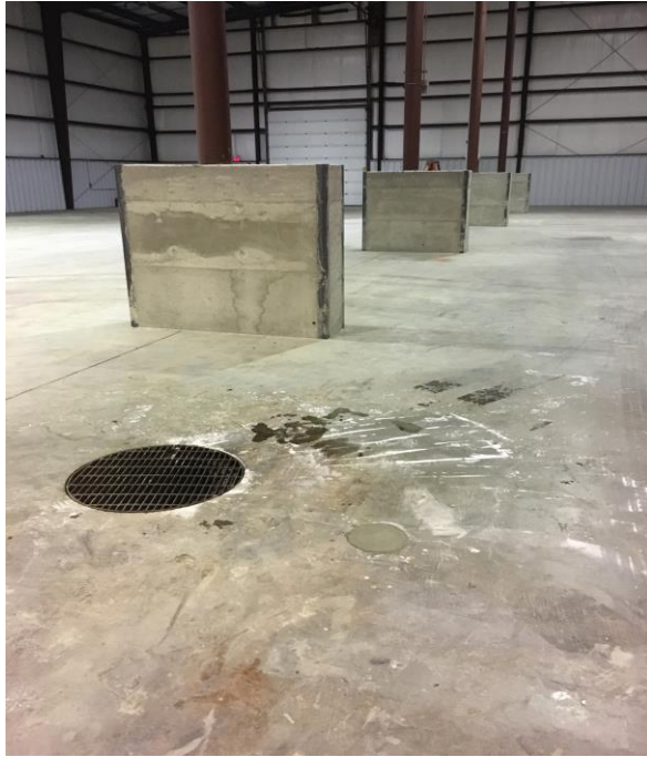
Photograph 1: Monitoring well TH19-11 inside building on site.
