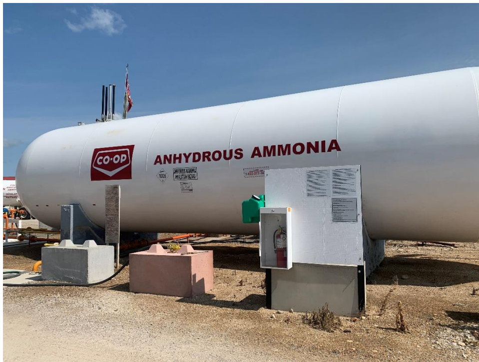
Photo 8 - 60 metric tonne tank containing anhydrous ammonia.
