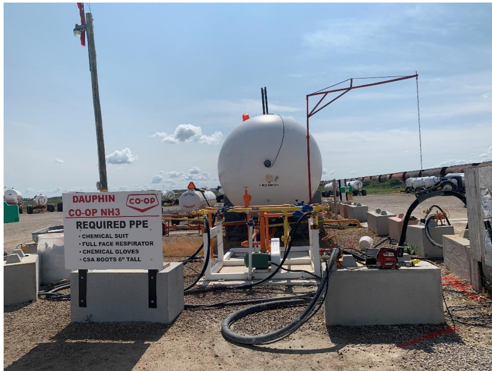
Photo 9 – Infrastructure associated with 60 metric tonne tank.
