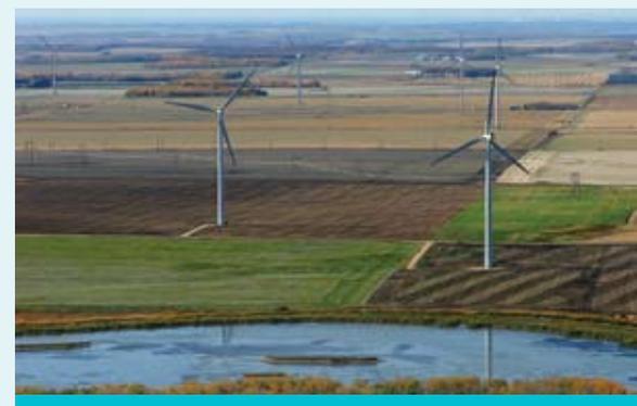
minute, a gearbox increases the speed so the magnets are spinning past the coils of wire more than 1,200 times per minute. Moving the magnets past the coiled wire causes electrons to move, creating electricity.
