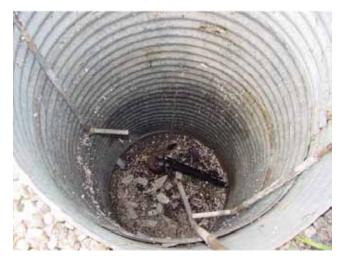
A **well pit** means a large diameter pit constructed below the ground surface for the purpose of housing a well. Prior to the mid-80s, it was common practice to construct a well pit around a small diameter well to provide winterized access to the well. This practice is no longer allowed for wells constructed for domestic purposes.
