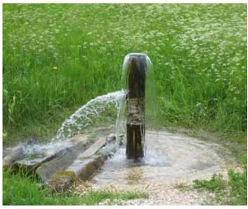
Flowing artesian wells must be sealed by a licensed well drilling contractor. The entire length of the well must be sealed using cement grout or a suitable mixture of sand-cement or bentonitecement grout.
