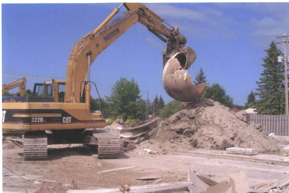
PHOTOGRAPH 3: Destruction of UST prior to loading into waste bin for transport.
