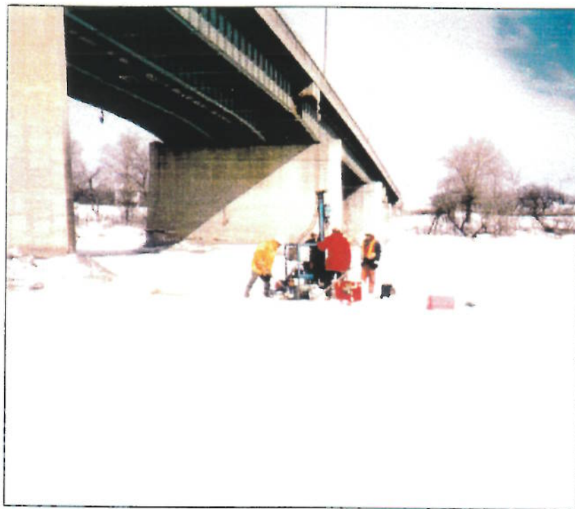
PHOTOGRAPH 1: VIEW OF THE DRILL RIG USED DURING THE INVESTIGATION DRILLING BH01-01 ADJACENT TO THE DISRAELI BRIDGE.
