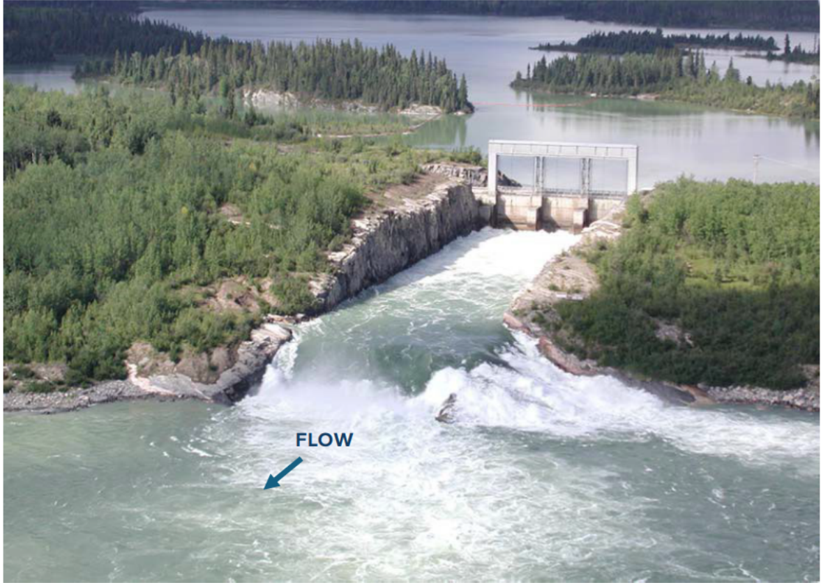
Figure 4 Photograph of Notigi Control Structure
