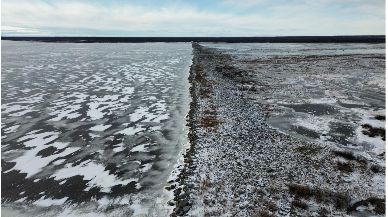
Figure 6 Photograph of the Churchill Weir
