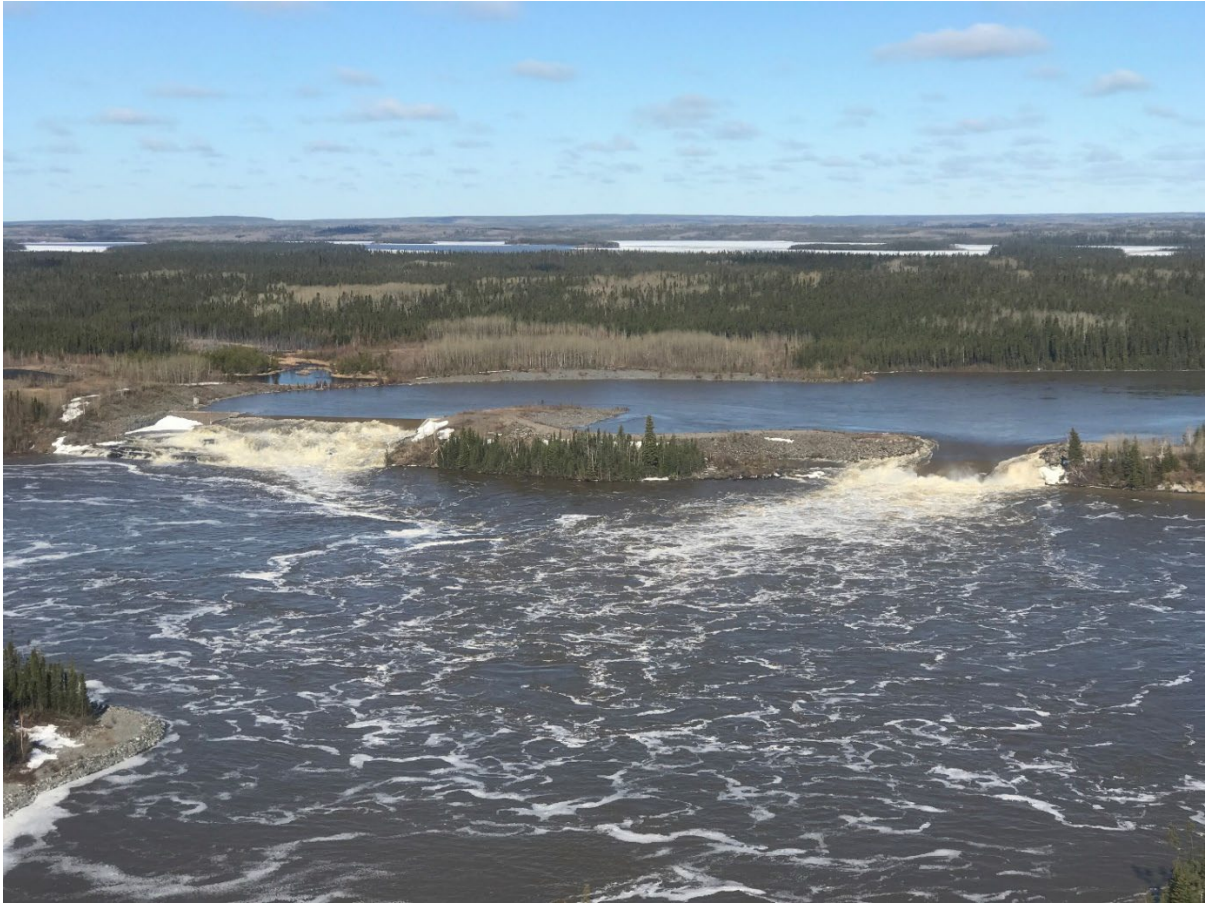
Figure 5 Photograph of Manasan Ice Control Structure
