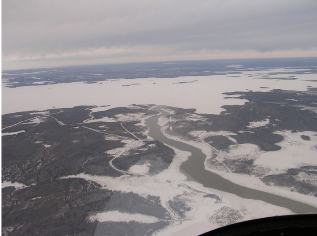
Figure 3 Photograph of South Bay Diversion Channel
