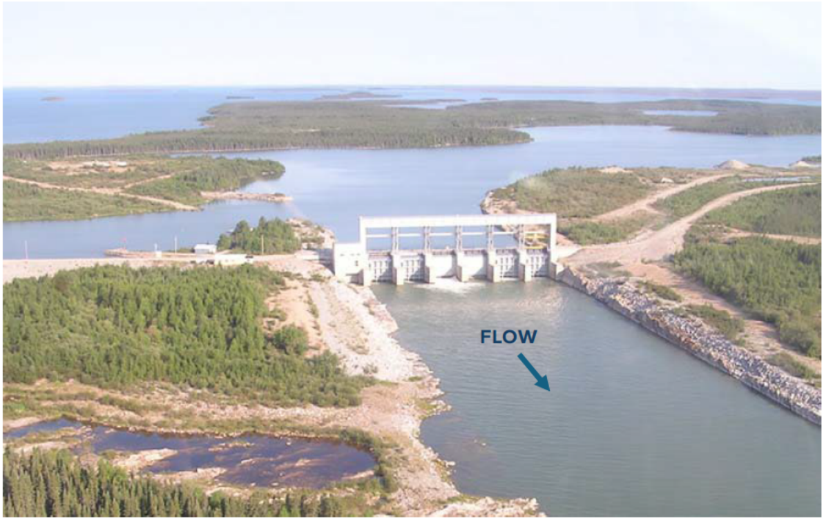
Figure 2 Photograph of Missi Control Structure
