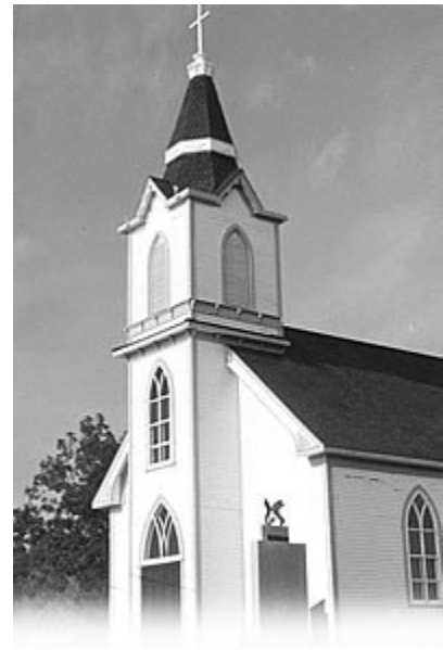
Hecla Church. Restoration complete 1973-1975.
